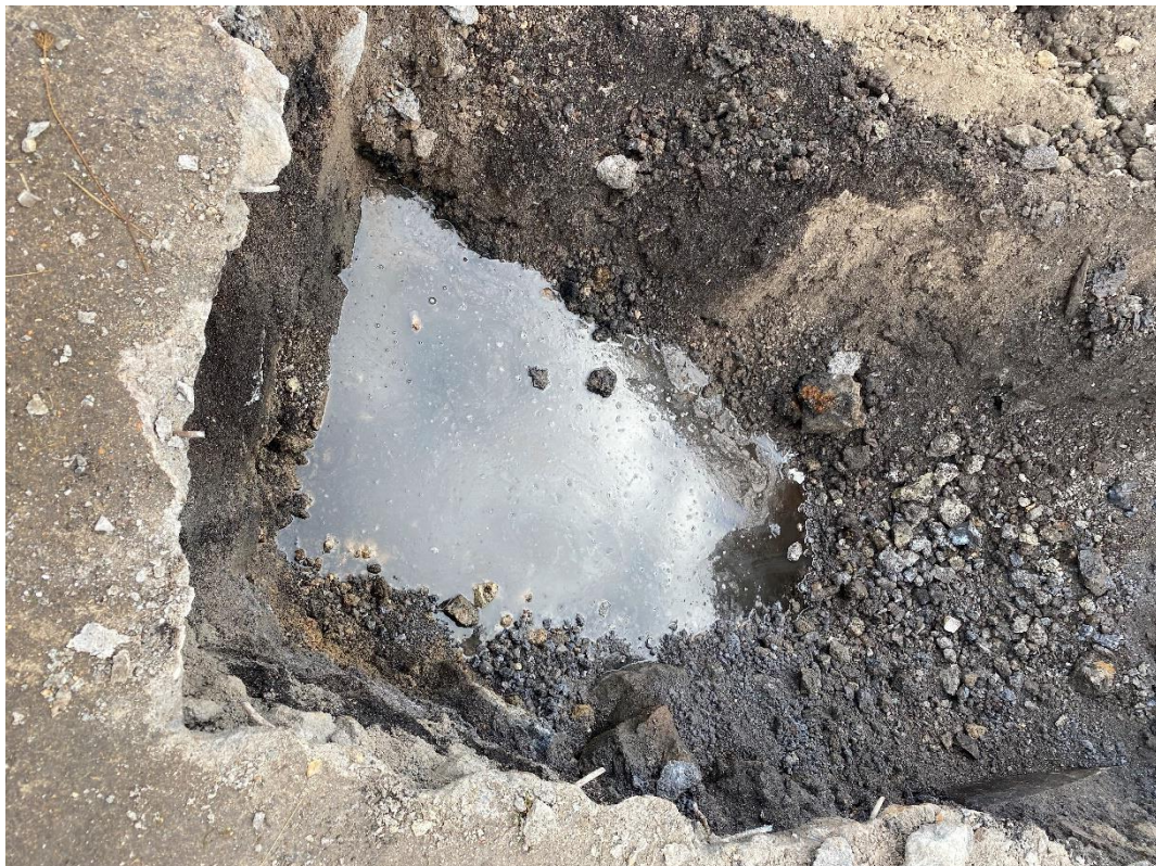
Photo 2: TP101 with groundwater resting at 1.5m bgl. (WSP, October 2020)
