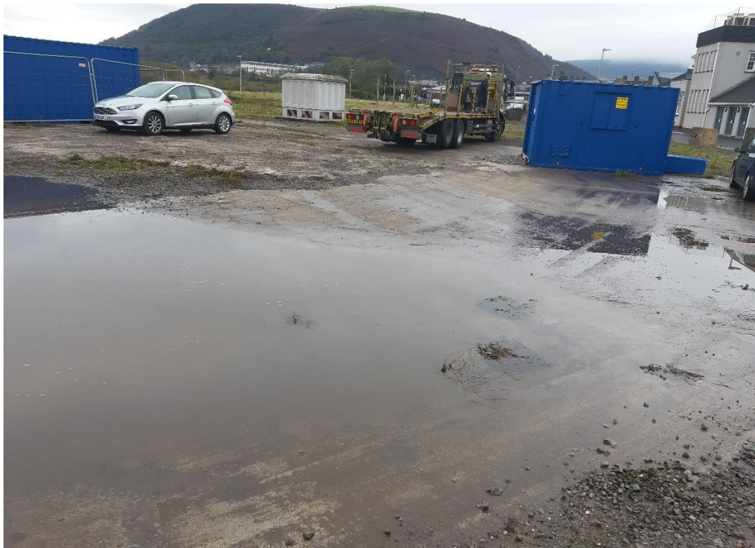
Photo 1: The gas holder base, view to the east. (WSP, October 2020)
