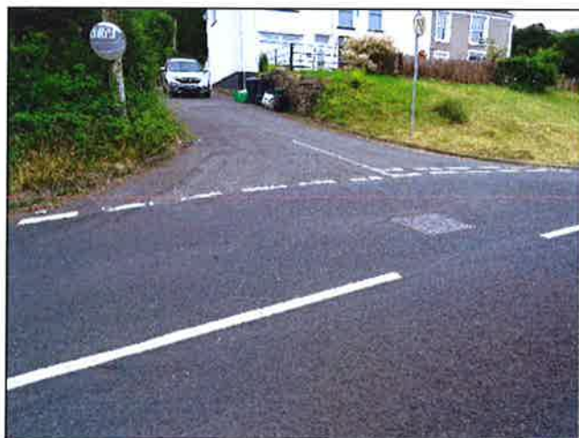
Access to Waterfall Road from B4434 Neath Road
