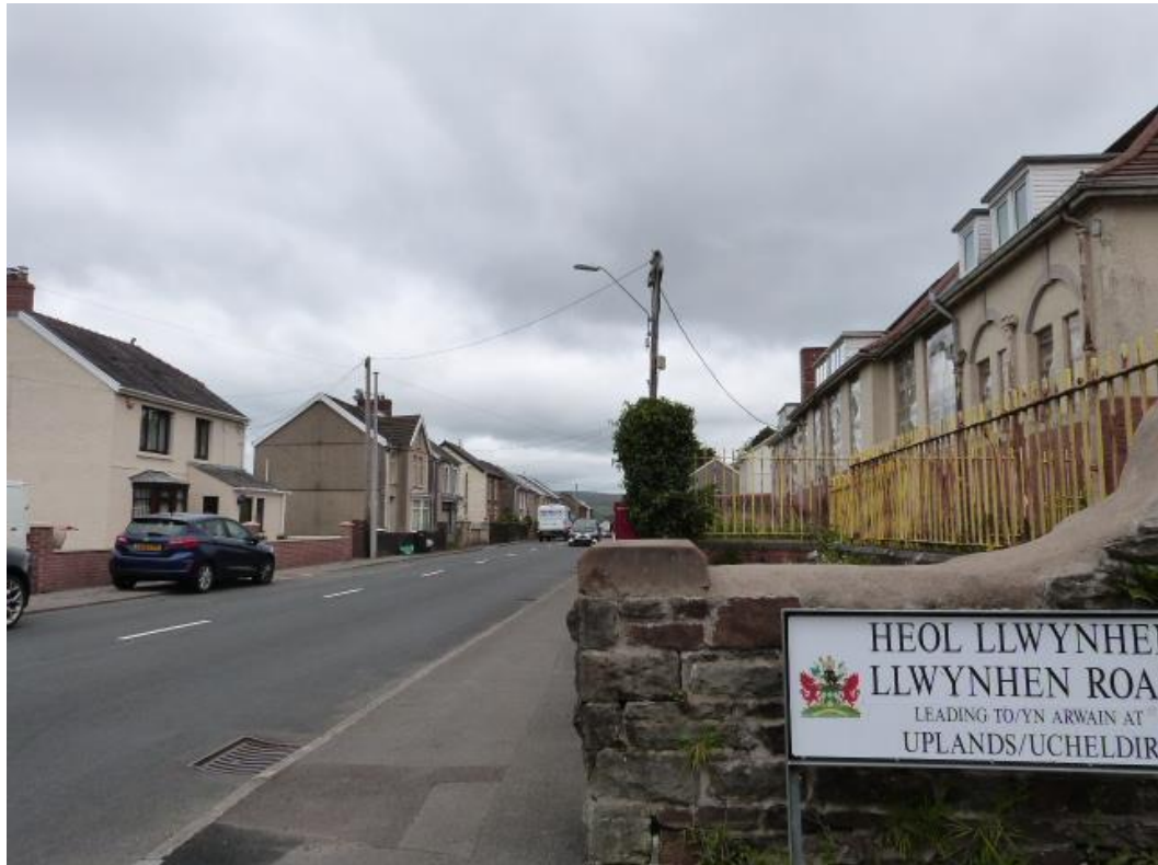
Plate 3: View looking north from access towards Gwaun-Cae-Gurwen
