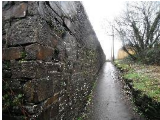
Plate 7: External view of West boundary
