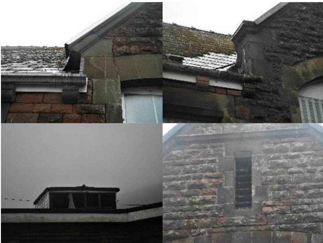
Plate 5: Potential access points to roof voids for bats
