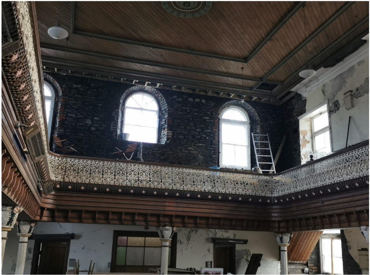
Figure 14 - Decorative, cast-iron handrails and ceiling
