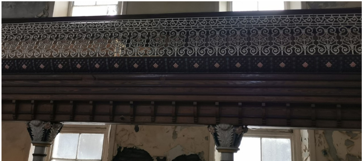
Figure 13 - Decorative, cast-iron handrails around the upper gallery of Bethel
