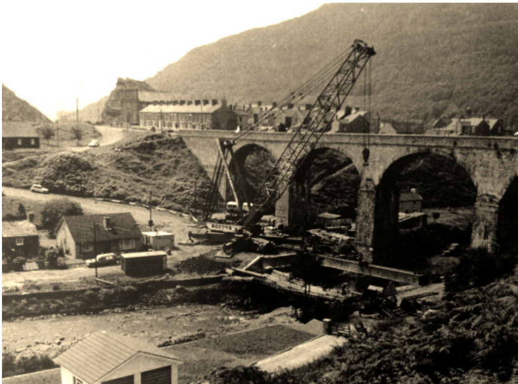
Figure 5 - The installation and construction of the new road bridge, near Dan-yBont in the 1960's
