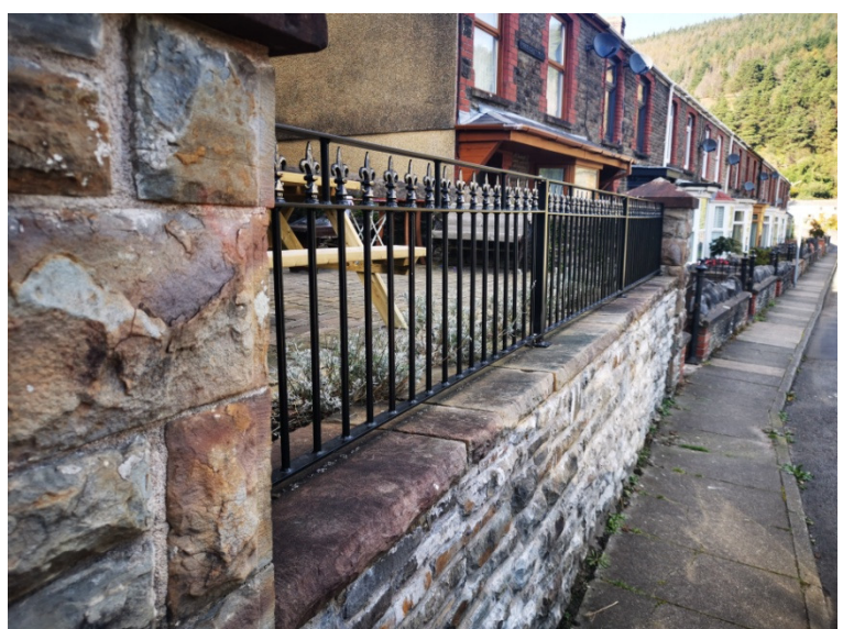
Figure 12 – Replacement railings, installed Dec'19
