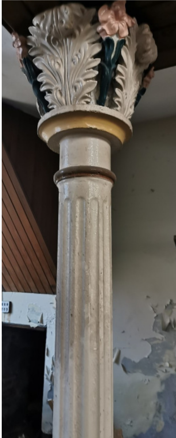
Figure 17 – One of the nine decorative, supportive cast-iron columns...
