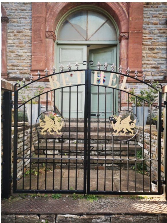
Figure 11 – Replacement gates, installed Dec '19
