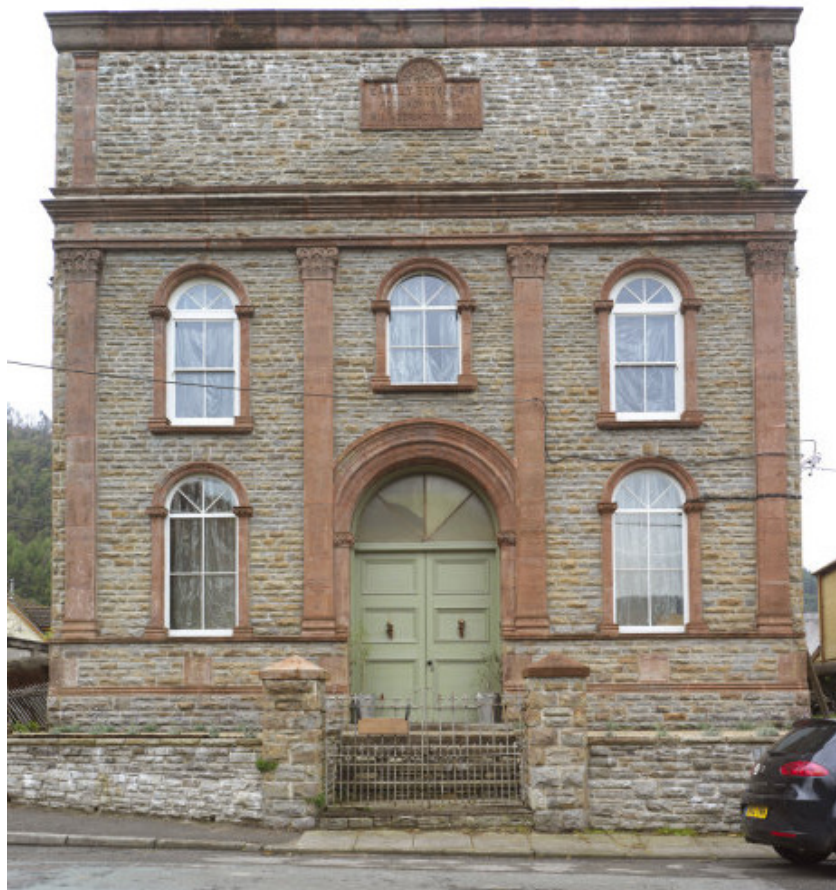
Figure 10 – Recently taken photograph of Bethel – the intention is to replace the damaged fanlight above the front door with stained glass, including the Burton name.
