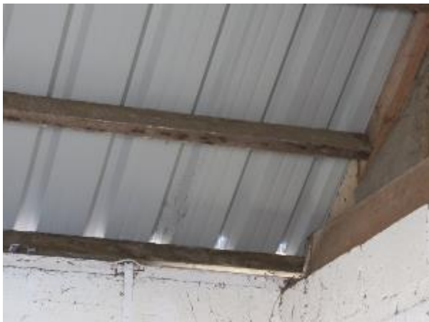
Photo 25: Gaps Under Ridges of Roofing Sheets
