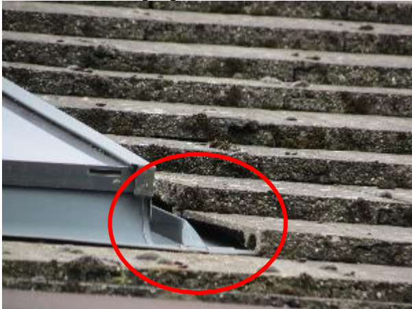
Photo 7: Eroded Cement Mortar Under Roof Tiles Near Solar Panel [R1]
