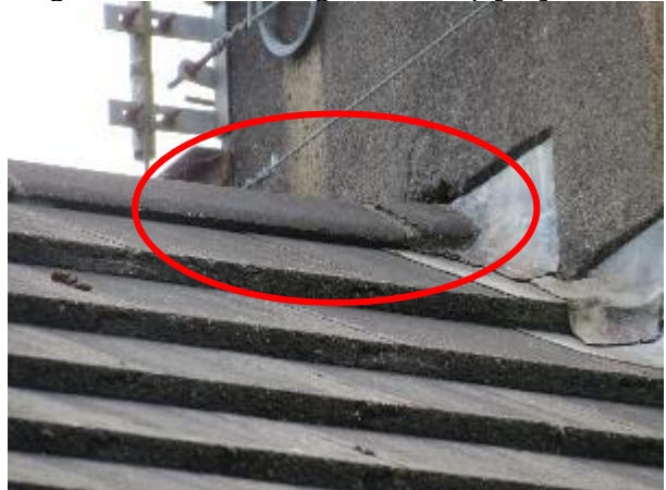
Photo 8: Gap Under Ridge Tiles and Gap Between Ridge Tile and Rendering of Chimney [R2]
