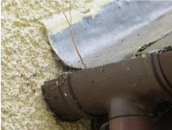
Photo 11: Gap Under Lead Flashing
