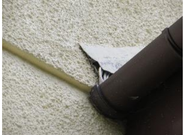
Photo 12: Cracked Soffit Box
