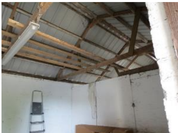
Photo 27: Roof Structure of Stables
