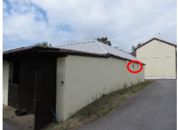
Photo 26: Dividing Wall in Poor Condition and Open Roof Void
