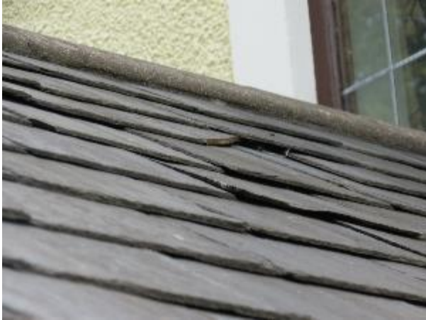
Photo 11: Gap Under Lead Flashing
