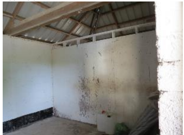
Photo 26: Dividing Wall in Poor Condition and Open Roof Void
