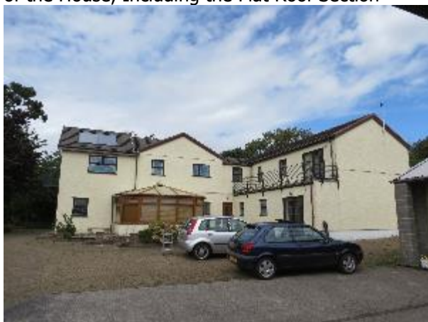
Photo 1: Southern and South-Western Elevations of the House, Including the Flat Roof Section
