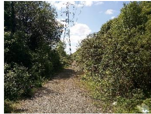
Site looking west from access gate
