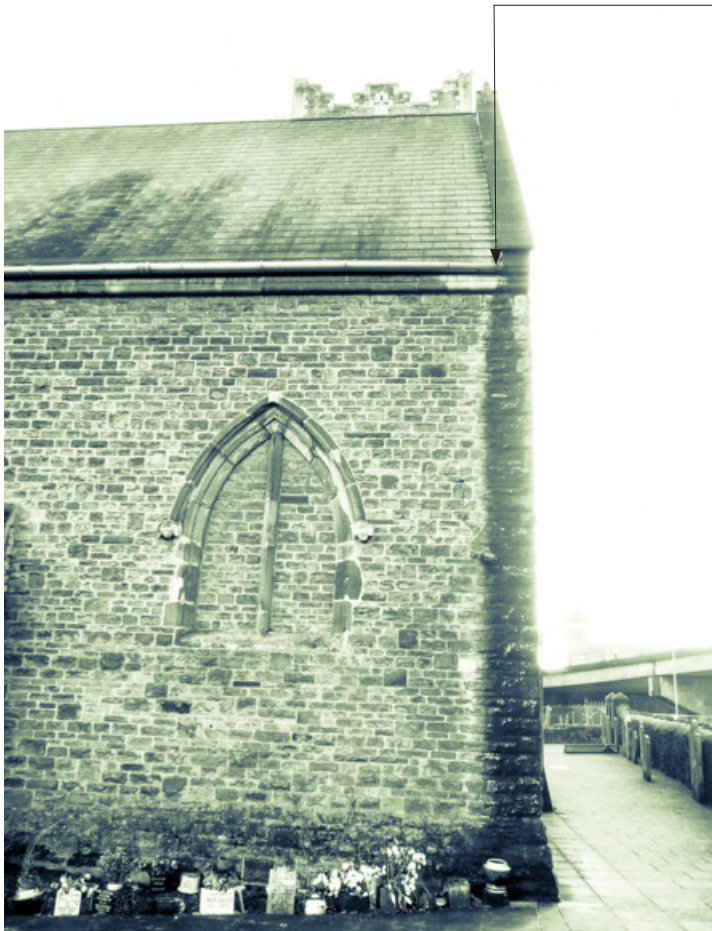
Image 402-03: North-west corner of the North Aisle
