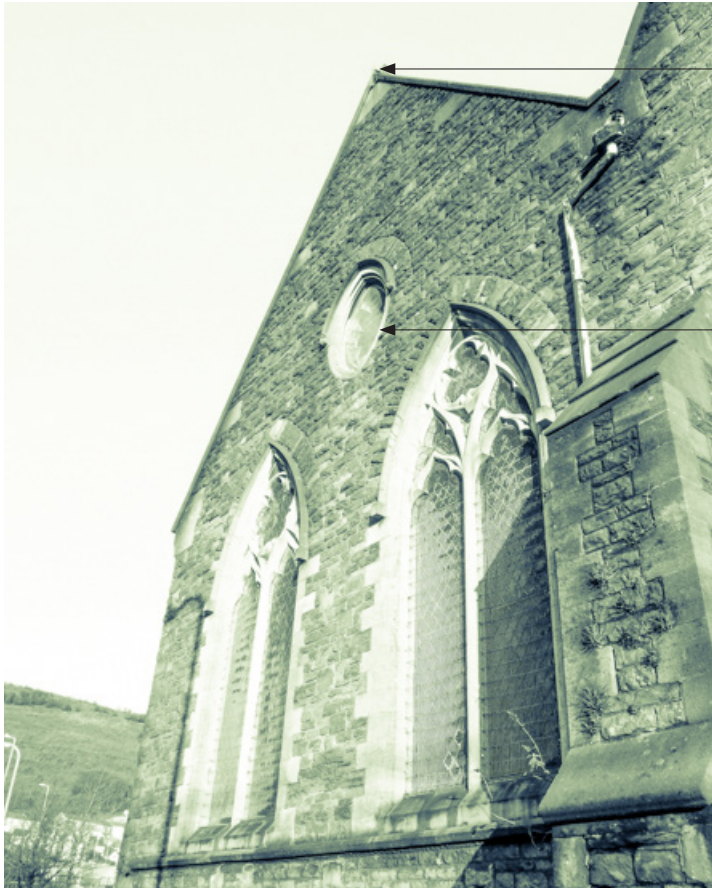
Image 402-01: West elevation of the North Aisle gable
