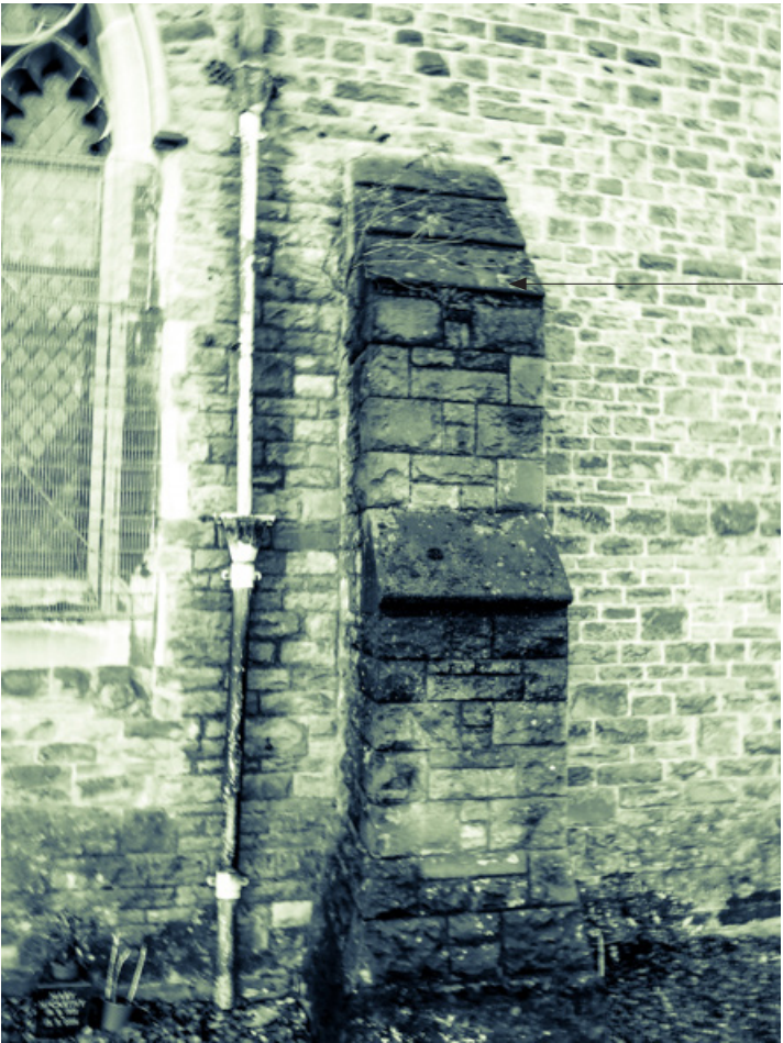
Image 402-04: Buttress to the North Aisle elevation
