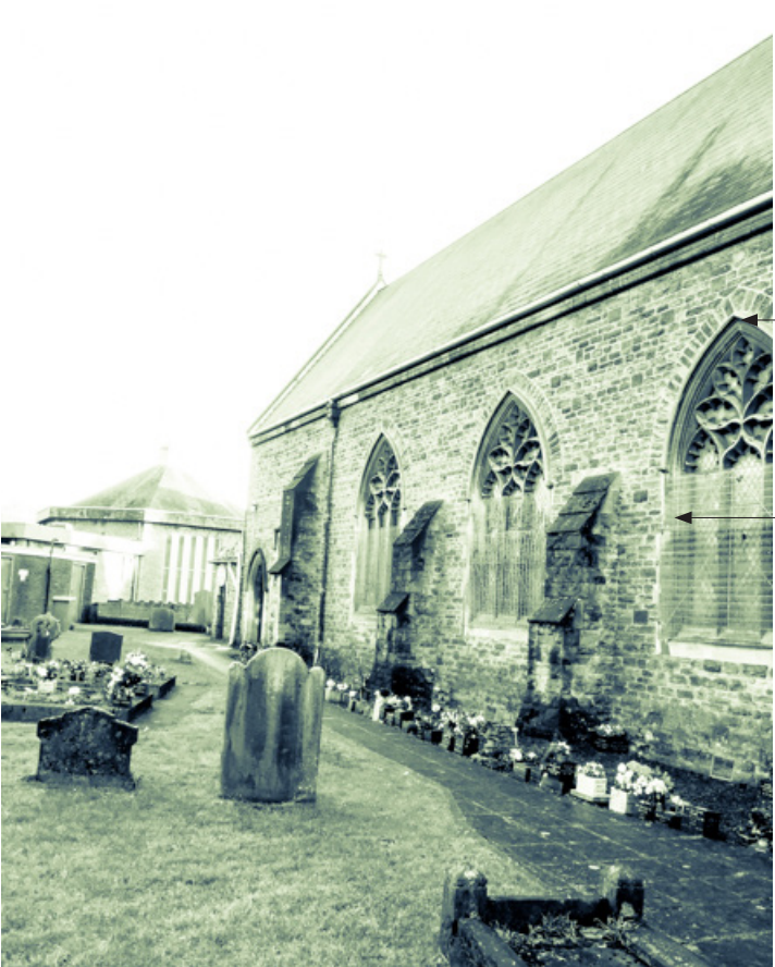
Image 402-02: North elevation of the North Aisle
