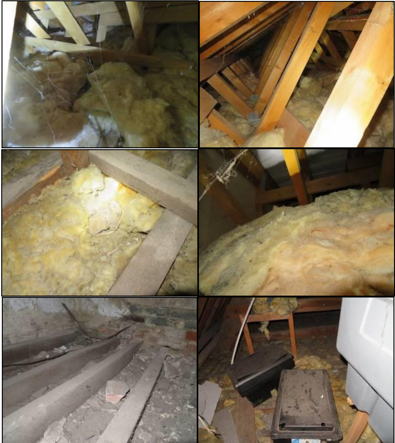
Additional interior images of the loft spaces at the annex property. There were many undisturbed cobwebs, a lot of dust, and some signs of rodent use but no bats or their signs were found.
