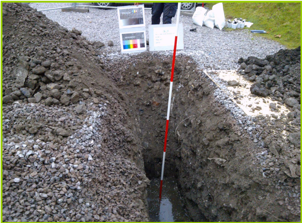
Plate 2: Trial Pit 1. Trial Pit sides.
