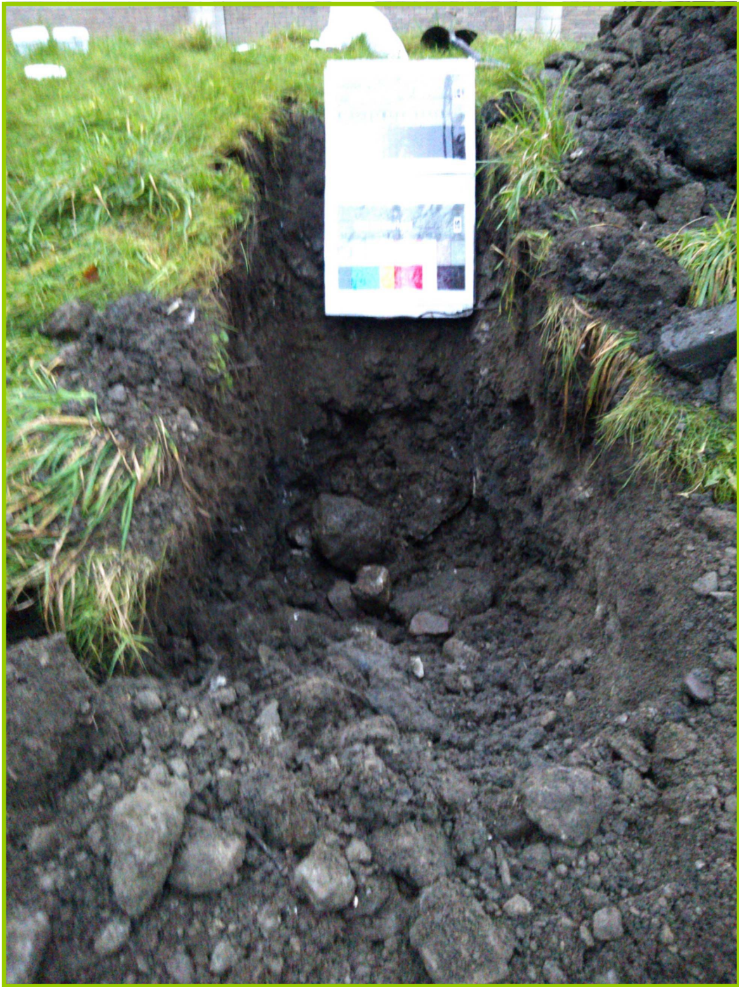
Plate 10: Trial Pit 5: Trial Pit sides.
