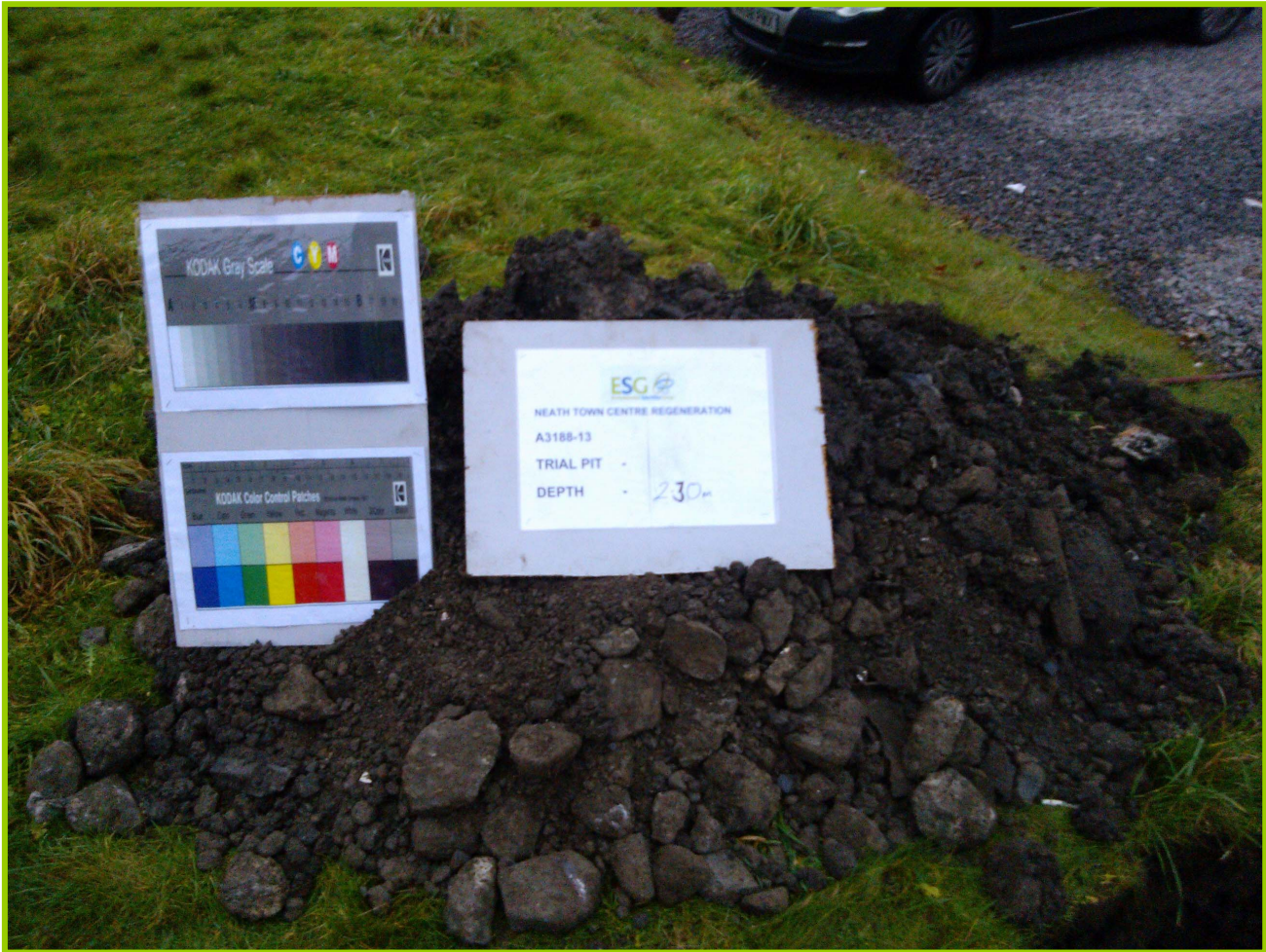
Plate 11: Trial Pit 5. Spoil.
