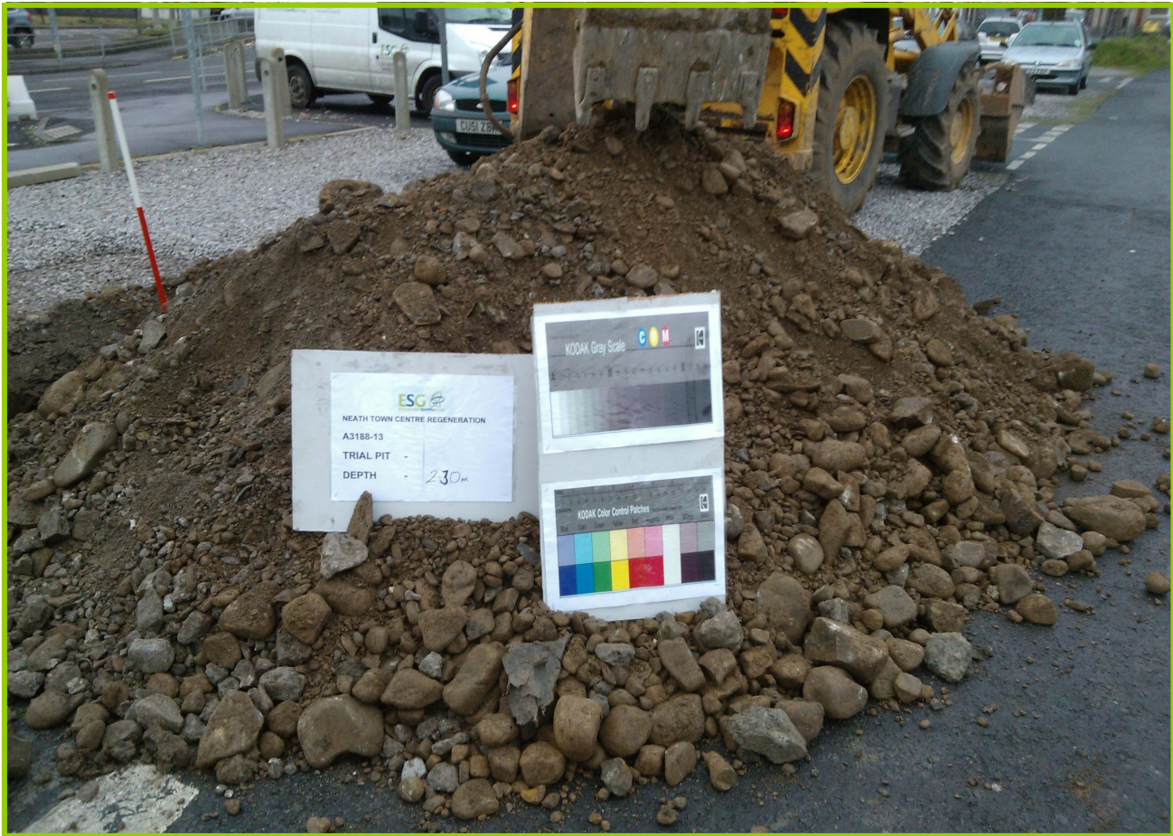
Plate 7: Trial Pit 3. Spoil.
