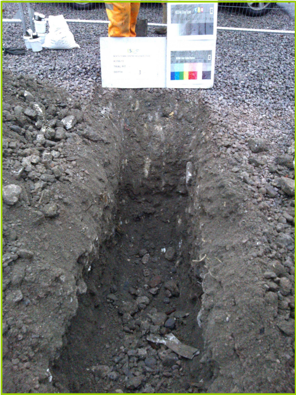
Plate 4: Trial Pit 2. Trial Pit Sides.
