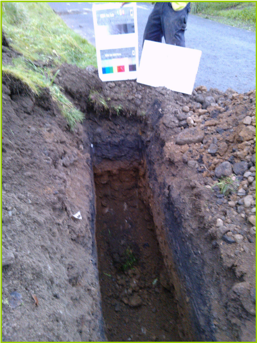
Plate 8: Trial Pit 4. Trial Pit Sides.
