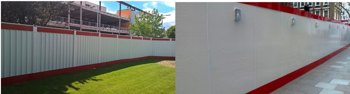
Example of replacement hoarding
