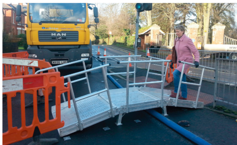
Pedestrian Ramp to Stores
