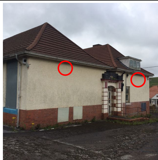
Figure 17. Bird box locations on north wall of main building.
