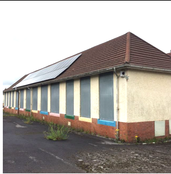
Figure 5. Main school building, eastern aspect.
