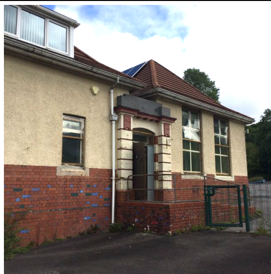
Figure 4. Main school building, southern aspect.
