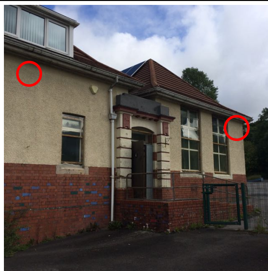
Figure 16. Bat box locations on south wall of main building.
