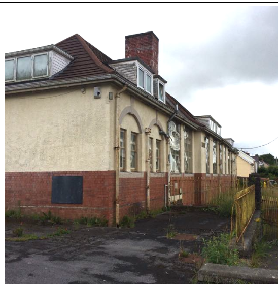
Figure 7. Main school building, western aspect.
