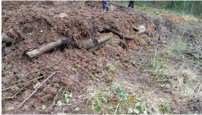
Photo 3. Hibernaculum in final stages of construction
