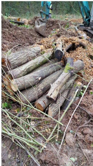
Photo 2. Logs being piled into the hibernaculum structure along with wood chippings.
