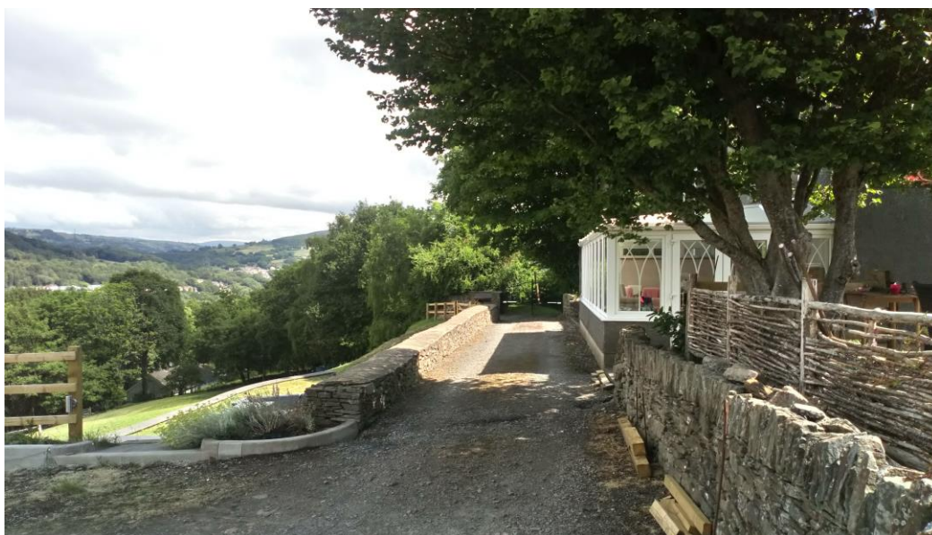
Image 3 – Illustrating existing private access track / driveway from Tramway Road across property frontage. Main access via black metal gates, with field access via existing timber gate (end of masonry wall).
