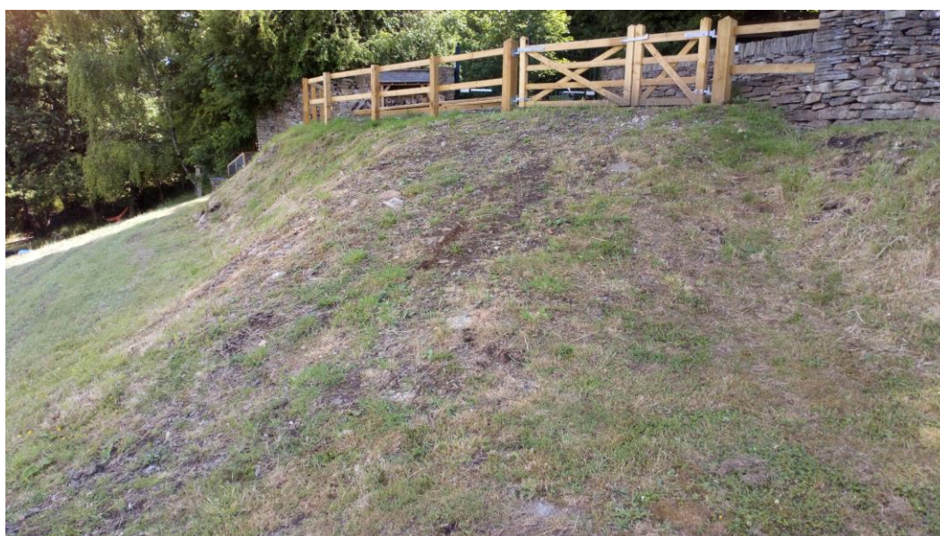
Image 4 – Illustrating existing grass sloped field access for quad (via timber gate), to remain unchanged.
