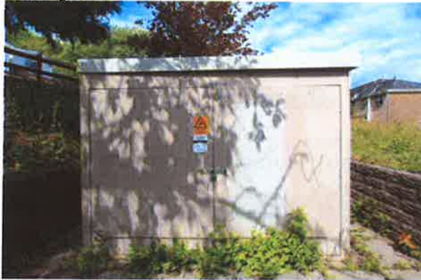
Photo 14: Single storey metal and glass fibre housing unit
