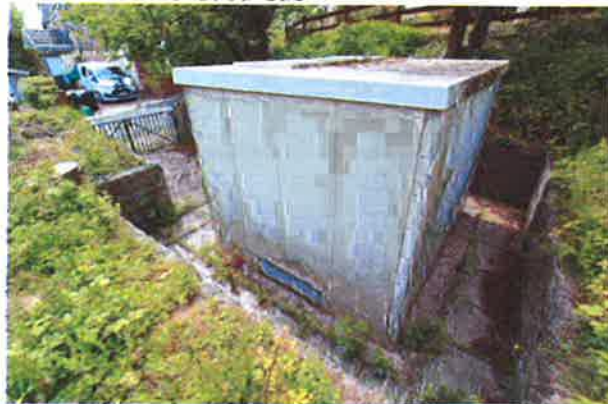
Photo 16: A retaining wall surrounds the structure, with access via Coed Cae
