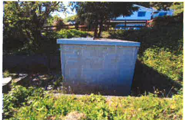
Photo 15: The structure is situated in a sunken compound
