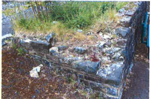
Photo 12: Crumbled cement and loose stones on the south-east boundary wall.
