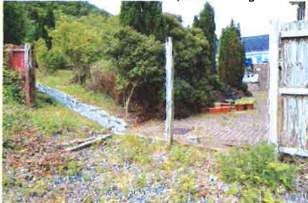
Photo 13: Section of wooden panel fencing removed
