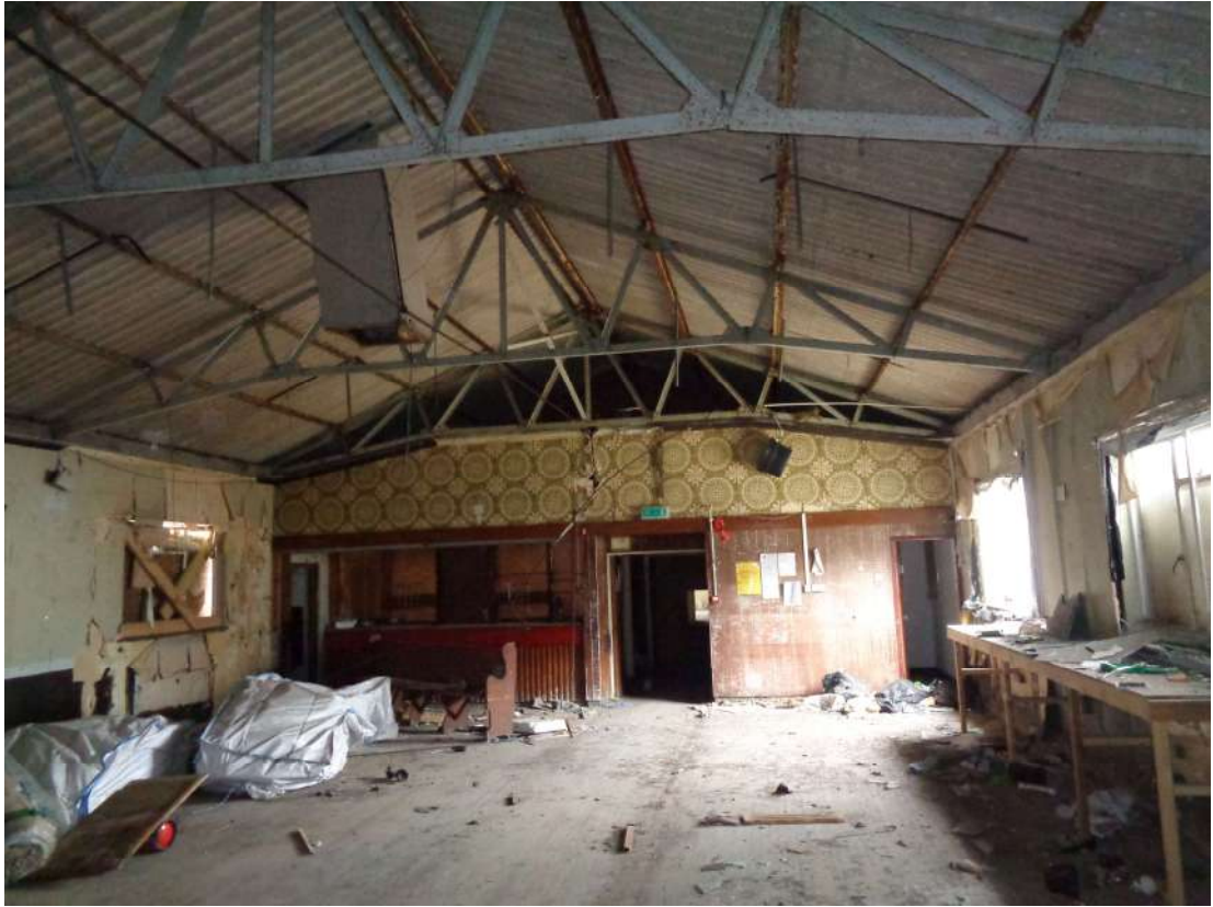
Photograph 5 – Internal view of workshop first floor level (facing front of workshop).
