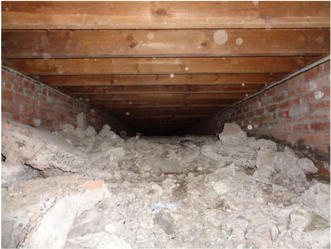
Photograph 7 – Sub-floor void beneath the majority of the workshop.
