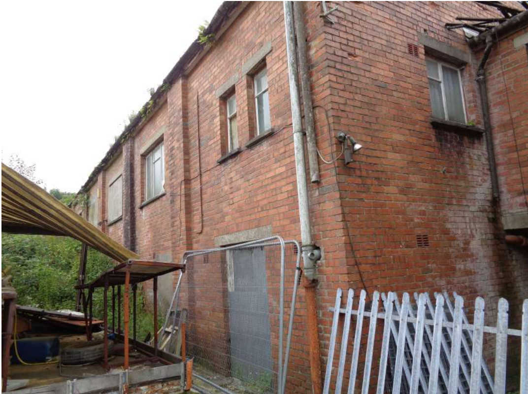
Photograph 1 – North wall of workshop.
