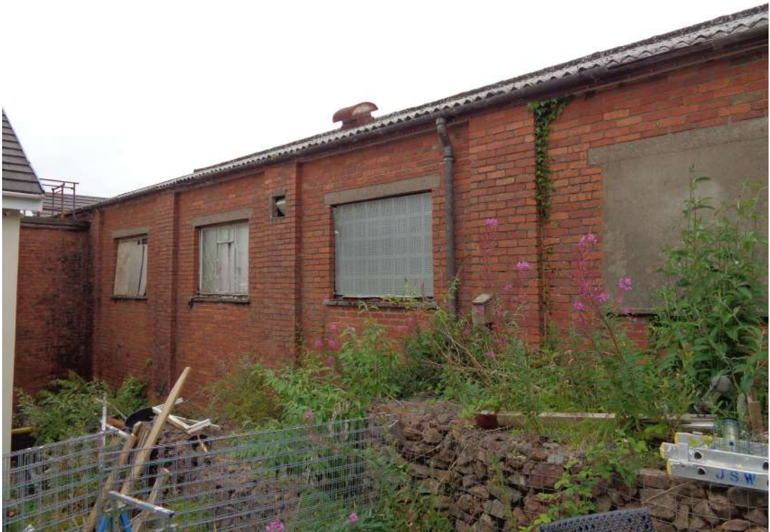
Photograph 3 – South wall of the workshop.
