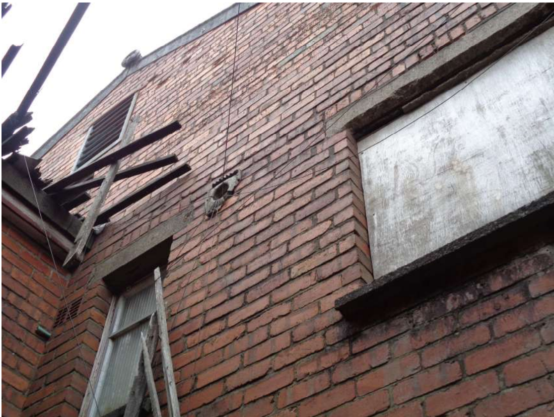
Photograph 4 – Front wall of the workshop.
