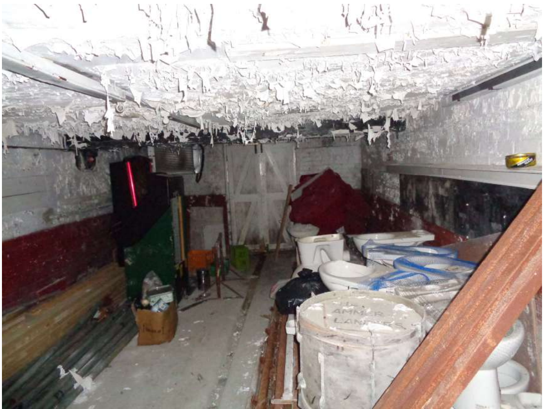
Photograph 8 – Main storage space beneath the area which is to be converted.
