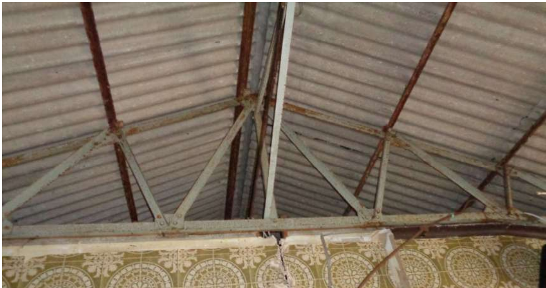
Photograph 6 – Roof truss on the line of the extent of the proposed conversion.
