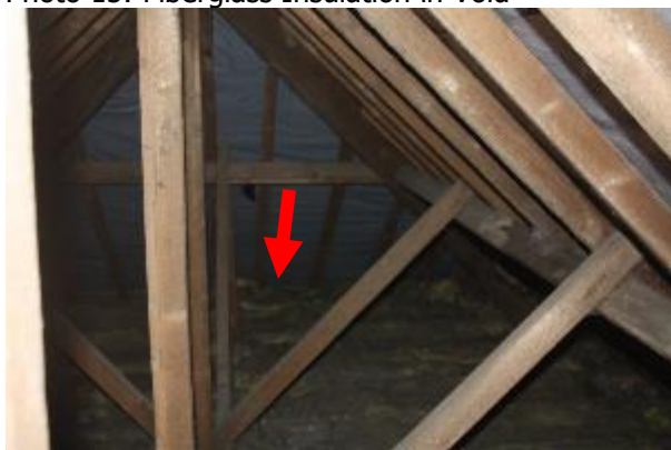
Photo 15: Fiberglass Insulation in Void
