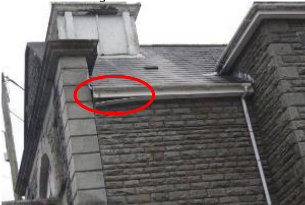
Photo 11: Damaged Soffit Box
