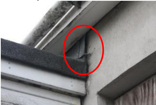
Photo 11: Damaged Soffit Box
