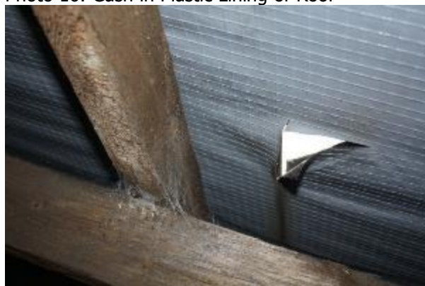
Photo 16: Gash in Plastic Lining of Roof
