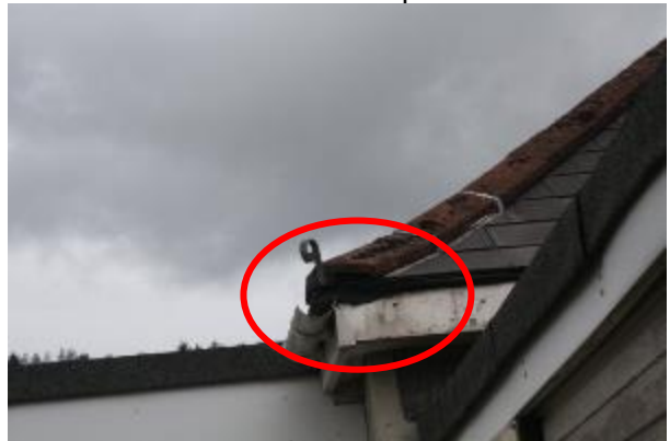
Photo 10: Access Via Broken Fascia
