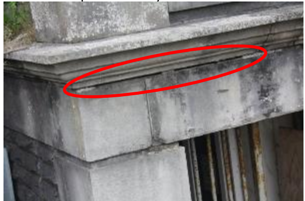
Photo 12: Gaps in Masonry
