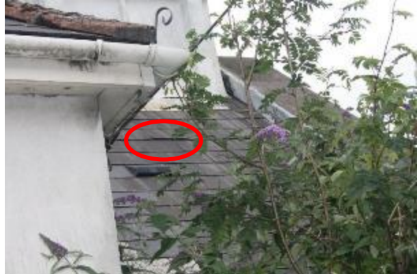
Photo 8: Eroded Cement on Hip Tile End
