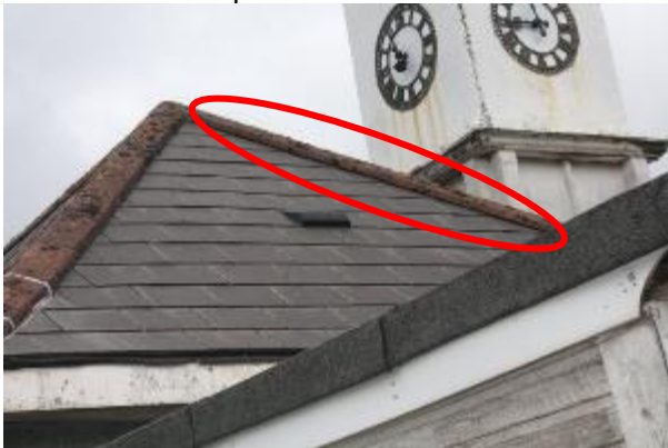
Photo 9: Gap in Bitumen Felt
