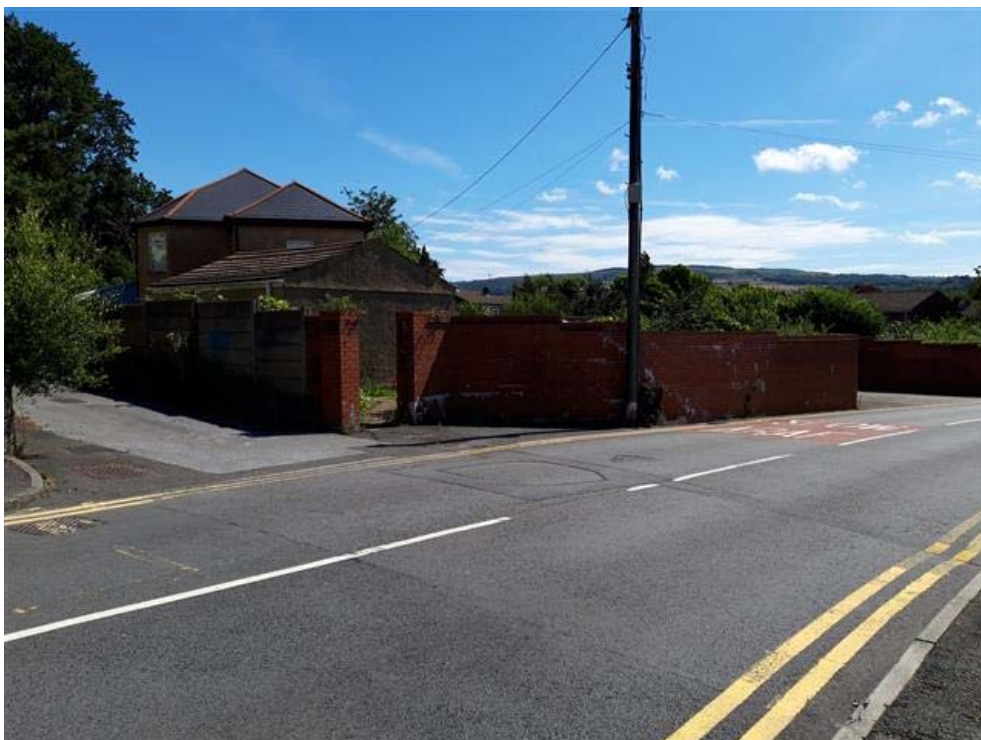
10. General view site boundary along Dwr-Y-Felin Road, and limited view of garage
