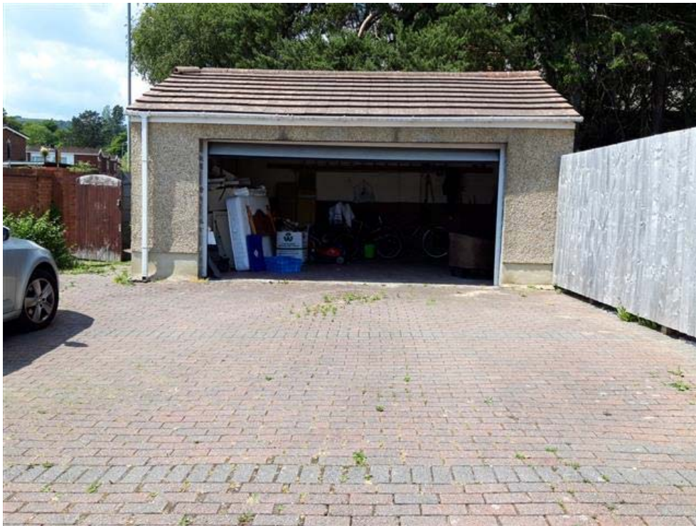
5. General view of existing garage (south elevation)
