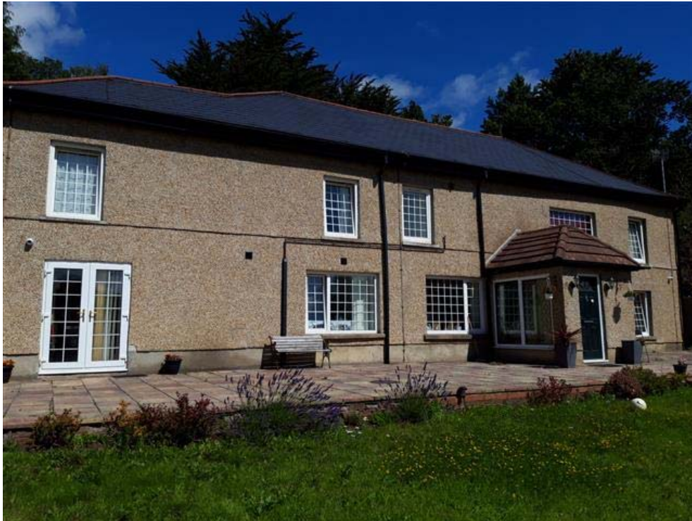
1. General view of the existing house (Front elevation)
