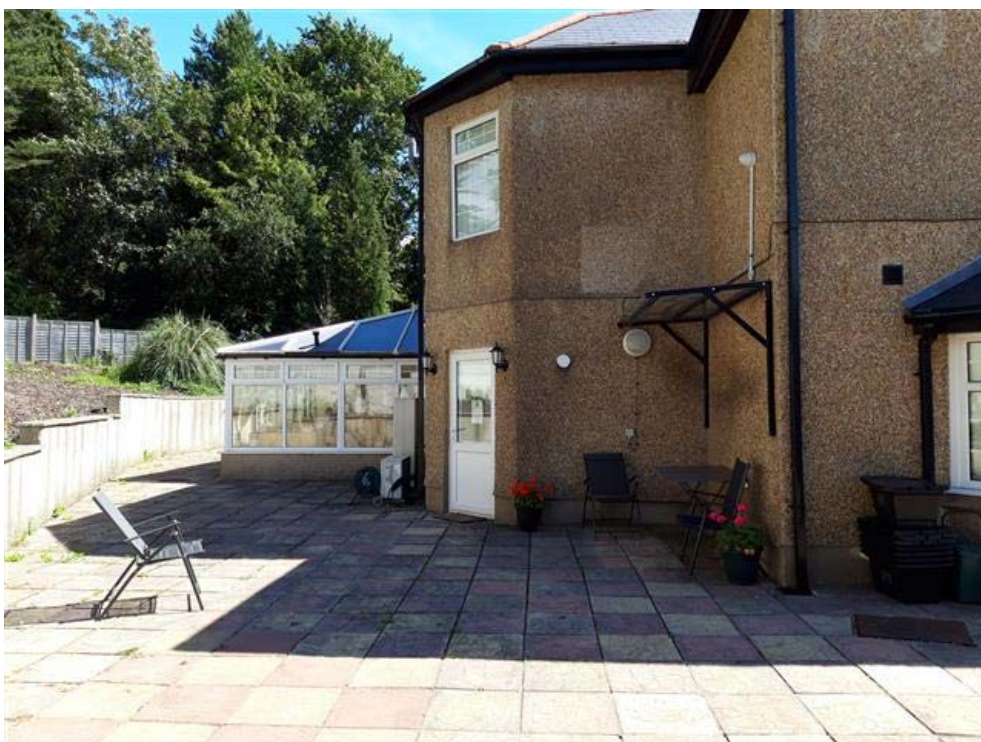
4. General view of house rear entrance from proposed flat entrance
