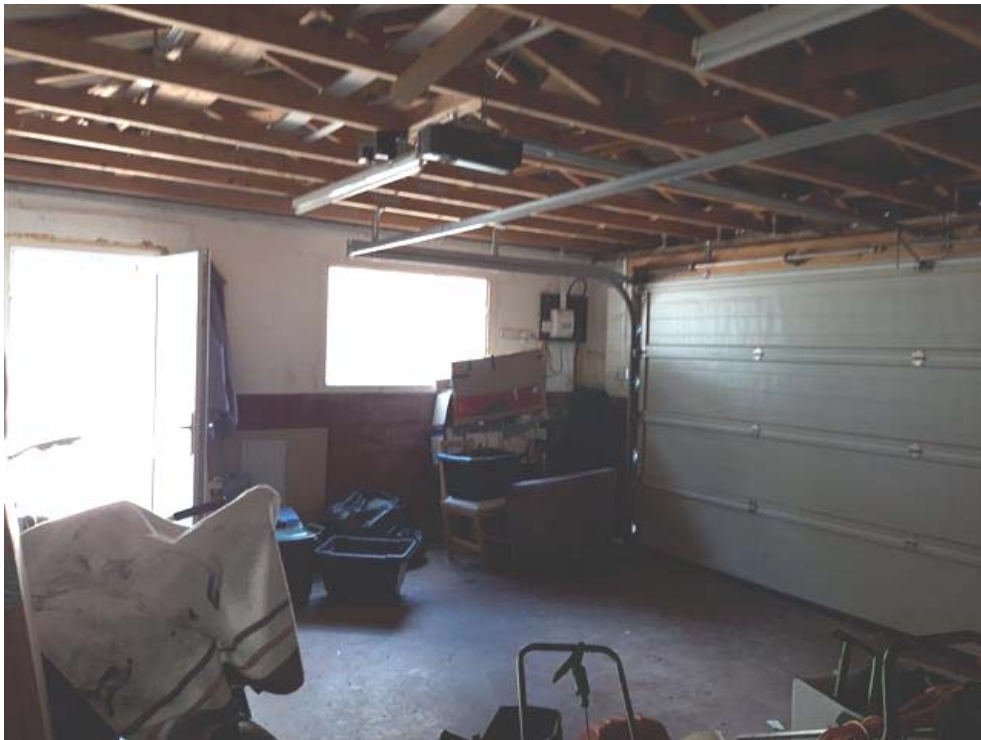
7. General view inside existing garage
