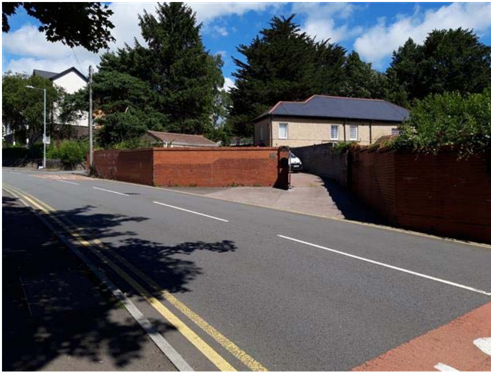
9. General view of site entrance and boundary wall along Dwr-Y-Felin Road
