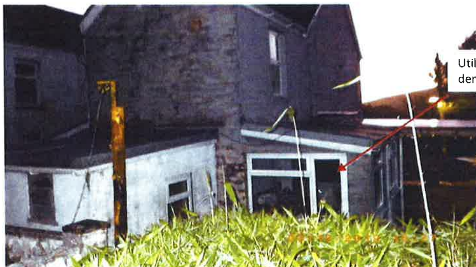
Rear elevation and Utility Room. The latter is to be removed.
