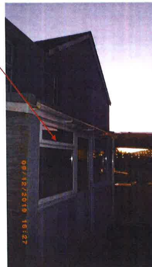
Utility Room to be removed.
