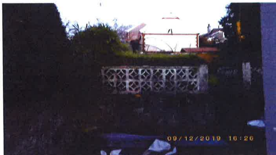
View looking at rear retaining wall and garden..
