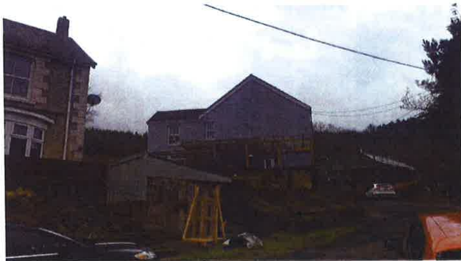
Side elevation & adjacent building/land.
