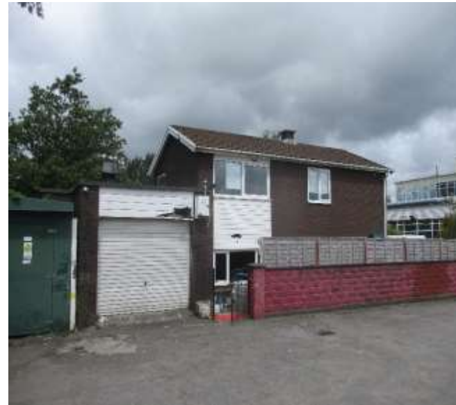
Caretakers House Rear Elevation Including Single Garage
