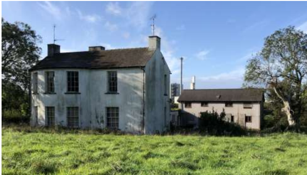
Photo 1 – view of the existing buildings at Tyn-y-Caeau
