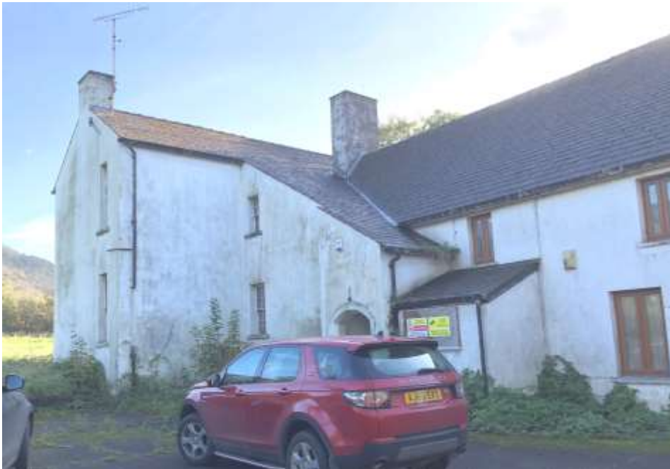
Photo 2 – view of side elevation of existing house
