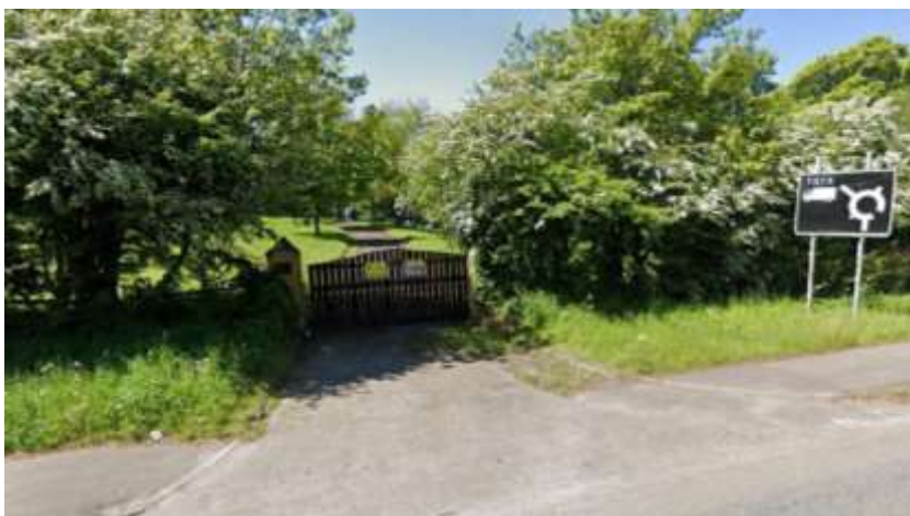
Photo 5 – existing access gates
