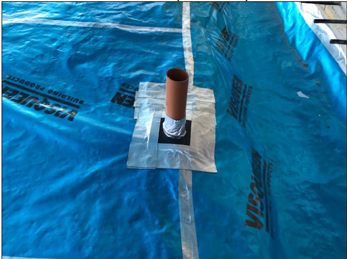
Plate26 Sealed Penetrations - (29/05/2020)
