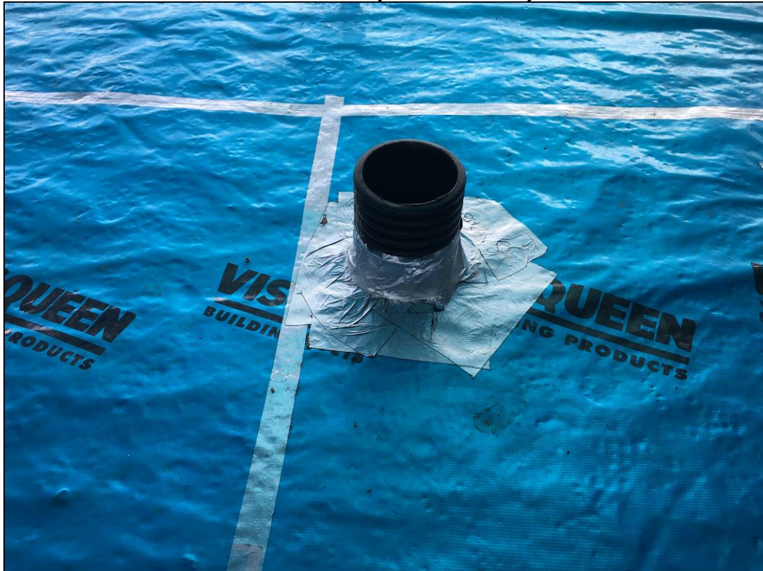
Plate 20 Sealed Penetration - (12/05/2020)
