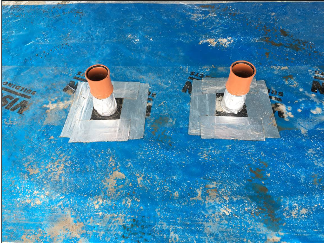
Plate 23 Sealed Penetrations - (22/05/2020)
