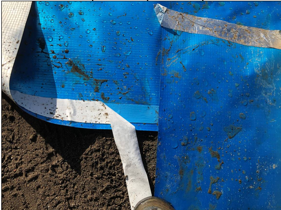
Plate 4 Double Taped Seams - (27/02/2020)
