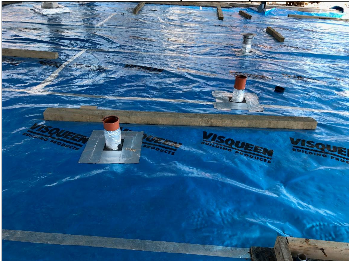
Plate 16 Sealed Penetrations – (22/04/2020)
