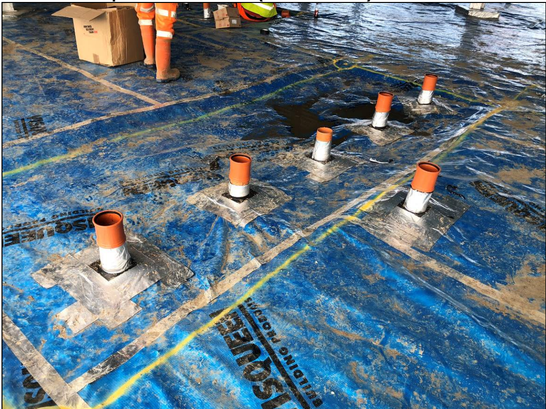
Plate 12 Pipe Penetrations - (08/04/2020)
