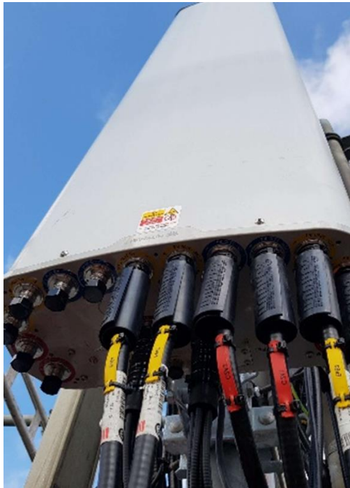
Source: Arqiva Trowell Services – 5G antenna and feeders
