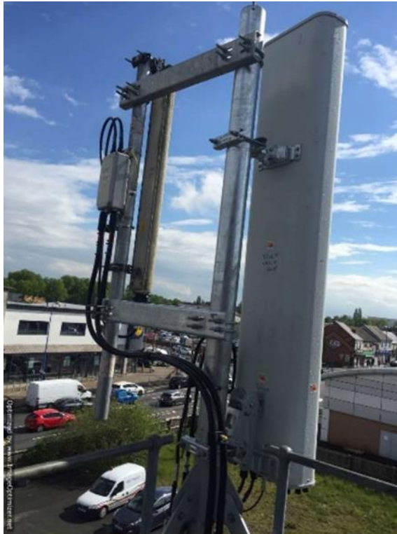
Source: Arqiva Blackheath Telephone Exchange – roof edge 5G antenna configuration
