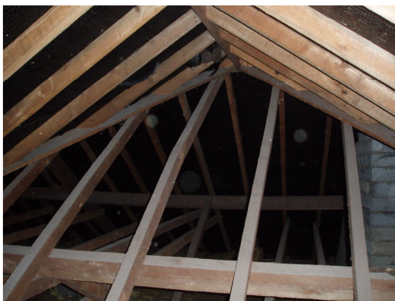
Looking from the loft over flat 6 to the main east west axis over flats 4 and 5
