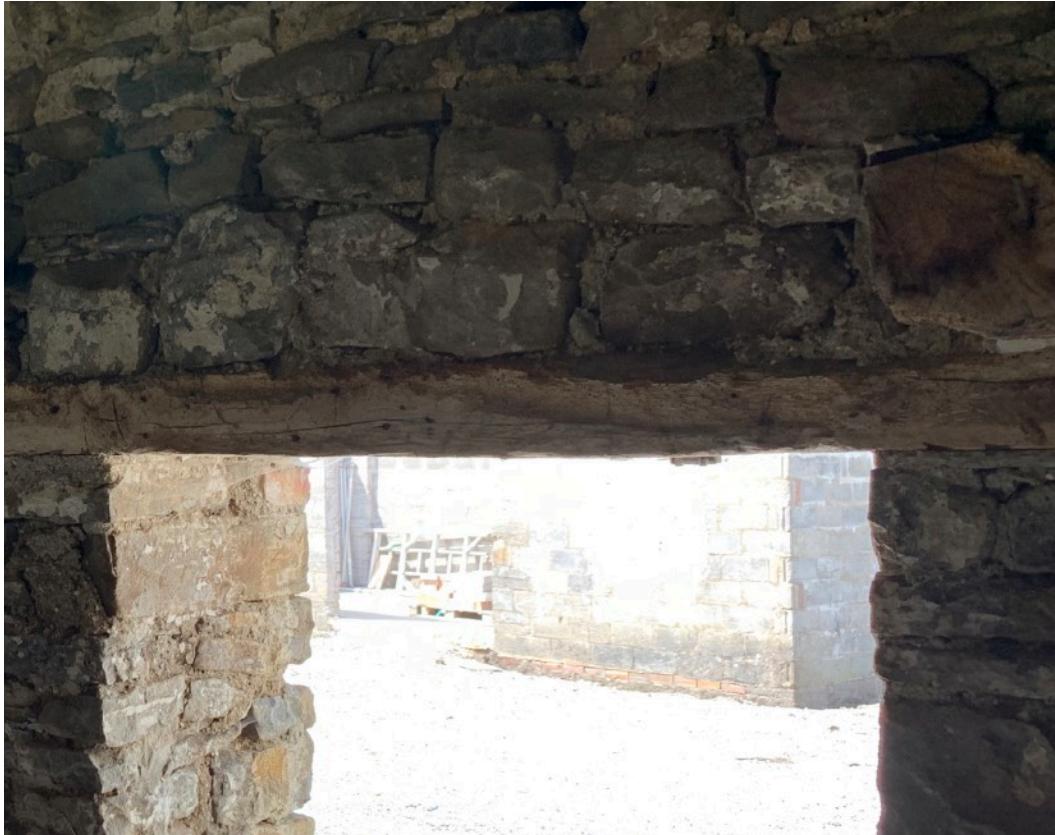
PHOTOGRAPH 4 TYPICAL EXISTING TIMBER LINTEL
