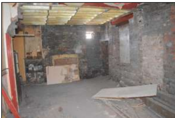
Photograph 5 – ground floor room in the single storey extension on the western side of the building. Showing access point to the interior of the building.
