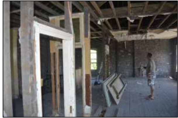
Photograph 2 – First floor of the building, taken from the southern end looking north.
