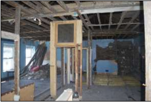
Photograph 1 – First floor of the building, taken from the northern end looking south.
