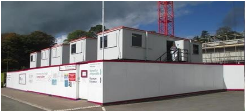
Typical site accommodation and welfare setup
