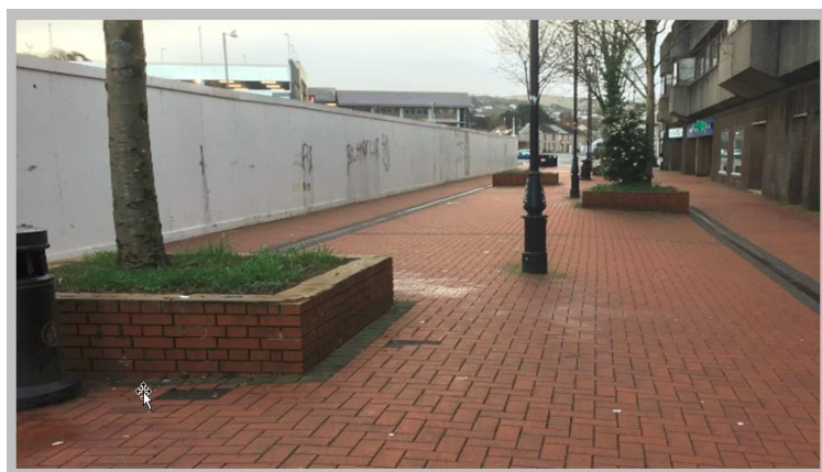
Perimeter Hoarding (re-positioned during the construction period) – Sequence (2)
