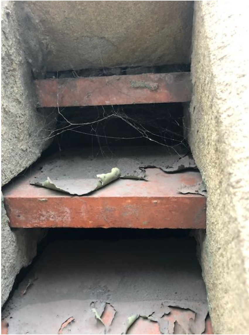
Louvered air vent under roof apex of porch
