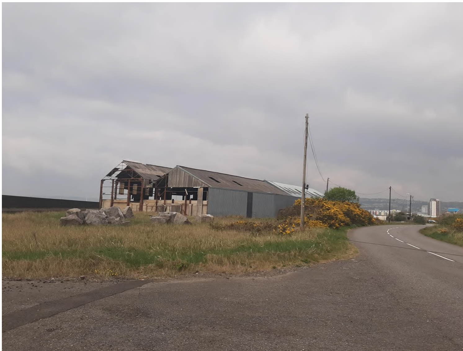
Photo of derelict building along the Western Landfall Area adjacent to Inset C (view – west)
