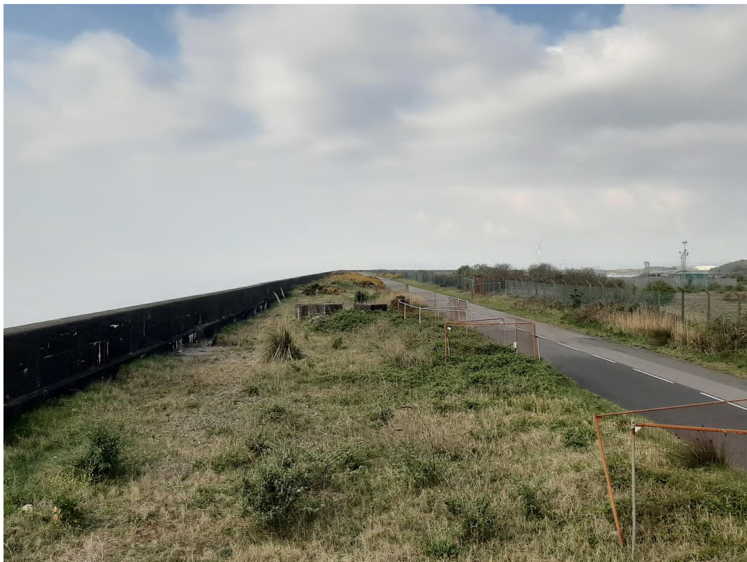
Photo along the seawall of the Western Landfall Access Road (view – south west)
