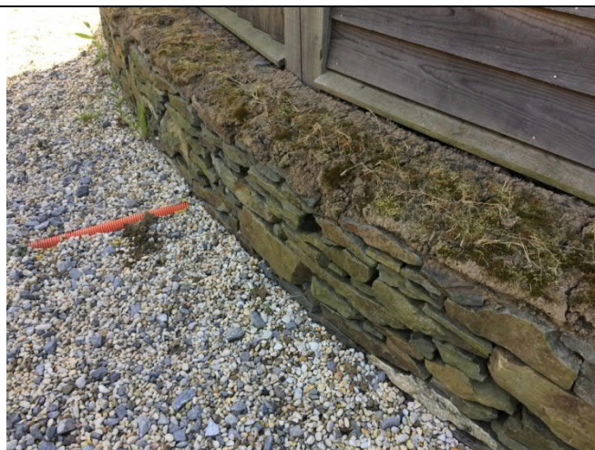
Photograph 11: Stone wall at the base of Building 2
