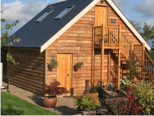
Larch cladding on Outbuilding
