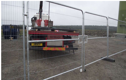
Figure 3.4 Heras Security Gates
