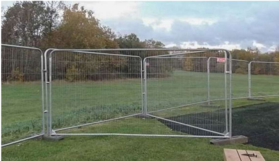
Figure 3.4 Temporary Heras fencing supports example.
