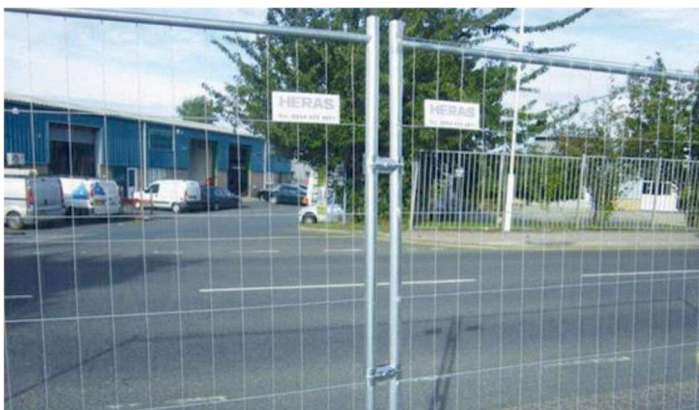
Figure 3.2 Heras fencing example
