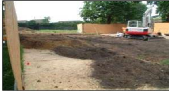
Ground protection image 2: Spreading soil excavated from footings is an effective way of buffering the plywood surface from the wear of light vehicles.
