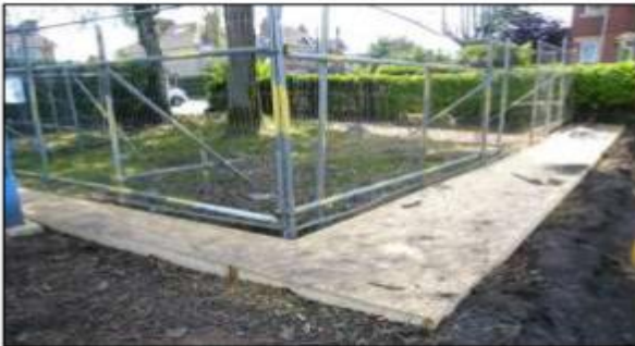
Ground protection image 3: Plywood fixed to a wood frame is another effective method of protecting soil from pedestrian compaction.
