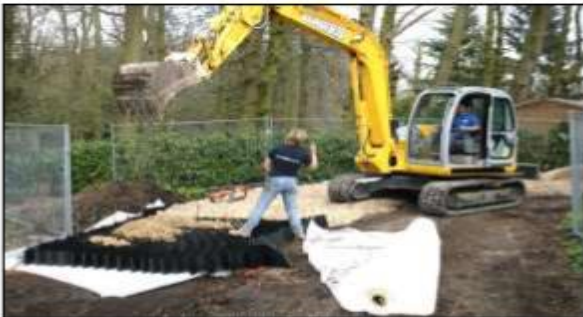
Ground protection image 5: Cellular products are a very effective means of providing ground protection where heavy vehicle use is expected. Here, it is being used to temporarily widen an existing road, to be removed once the construction is finished.
