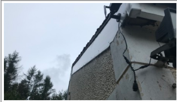
Photo 1: South-east facing gable end
