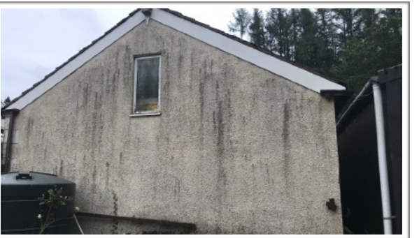
Photo 8: North-west facing gable end
