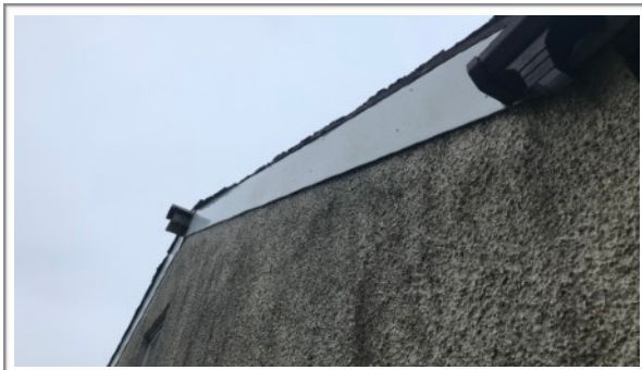
Photo 5: South-west facing gable end
