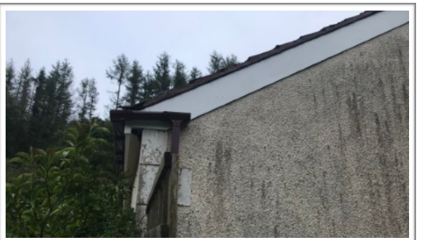
Photo 4: View of the roof/fascia interface
