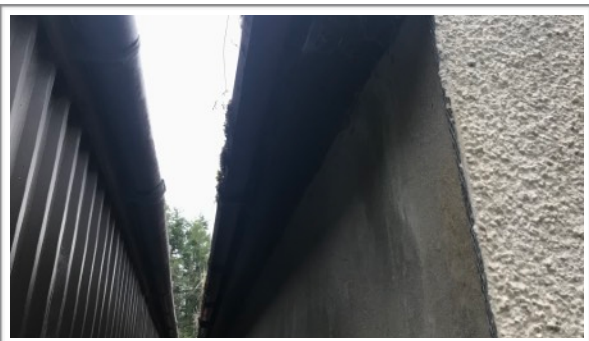
Photo 3: South-west facing elevation
