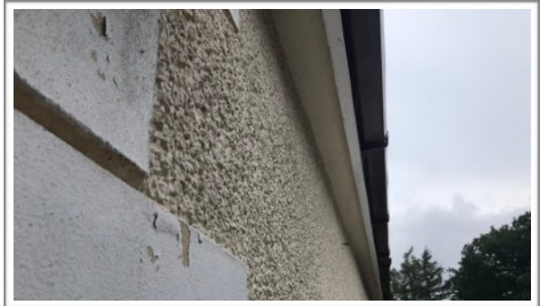
Photo 2: North-east facing tight soffits/fascia boards
