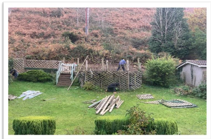
Right; Previous decking structure in the process of being removed.
