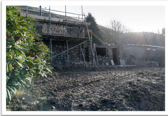
Left: Photograph looking east from adjacent to the boundary with Dan y Ffynnon House and looking at the currently partially completed outbuilding. With the 1 st floor summerhouse element removed, the single storey garden store and patio are of comparable height to the neighbours' outbuilding.
