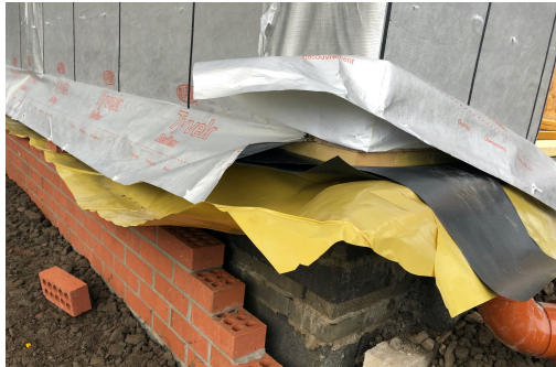
Images showing the installation of the radon barrier
