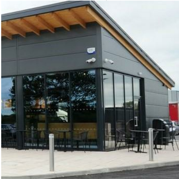
Composite Panels Cladding To Match Roof Colour
