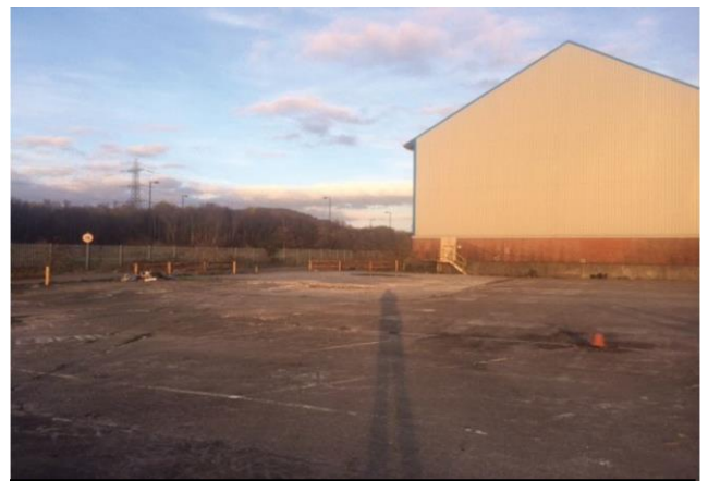
View from West – Car park and gable end
