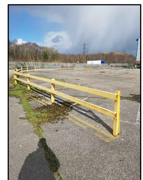
Image A:A - Existing Site Fence
