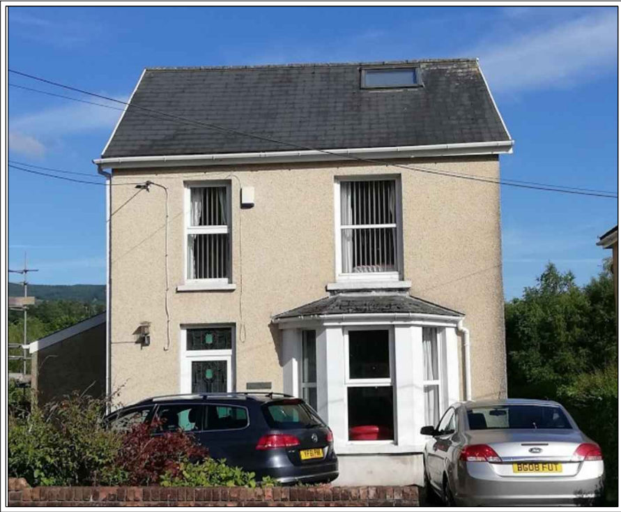
Photograph showing front elevation No changes caused by proposals
