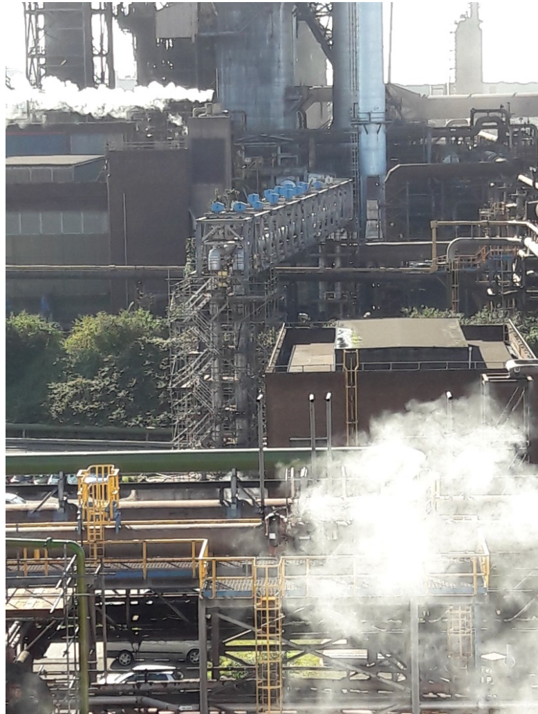
Figure 3.2: View of Bridge from Scaffold Tower at Margam C looking South towards the Bridge
