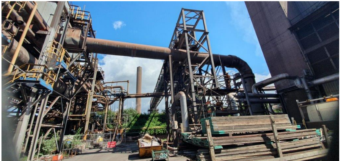
Figure 5.1: Image taken from ground level at the South end of the Bridge, looking North
