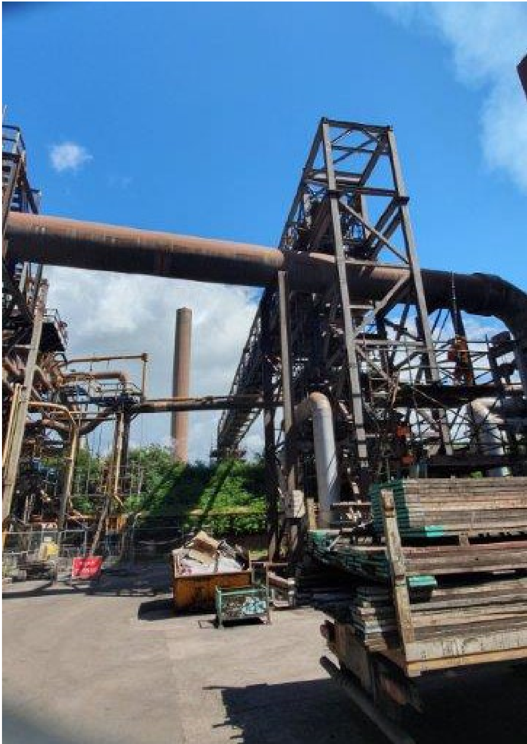
Figure 1.9: Ground level at the South end of the Bridge, looking North
