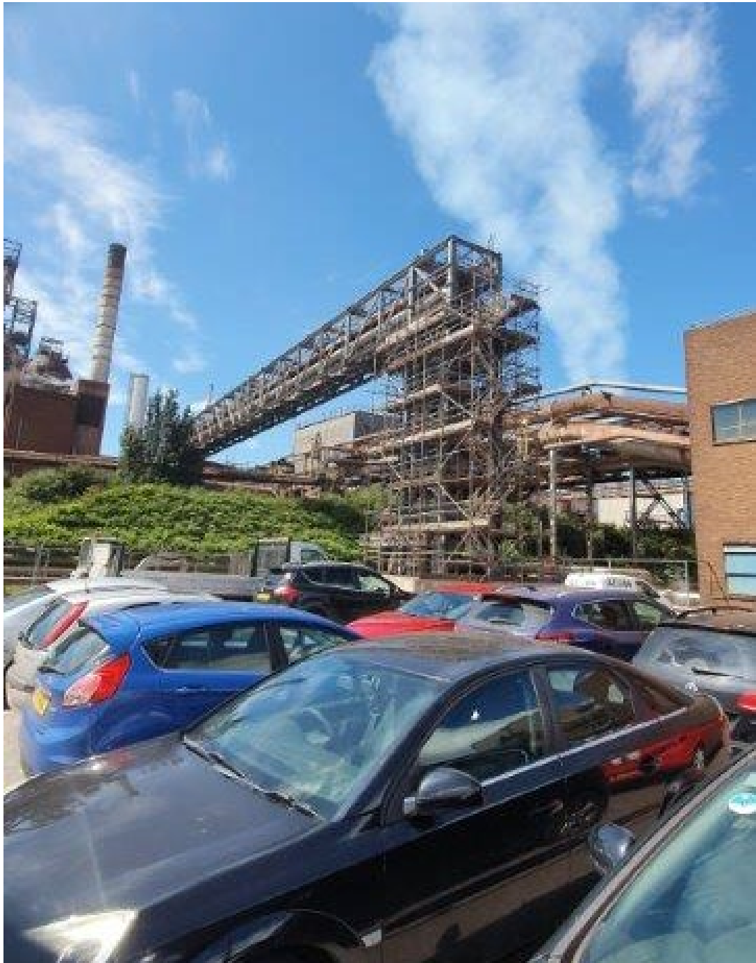
Figure 1.6: Ground level, North of the Bridge, looking South
