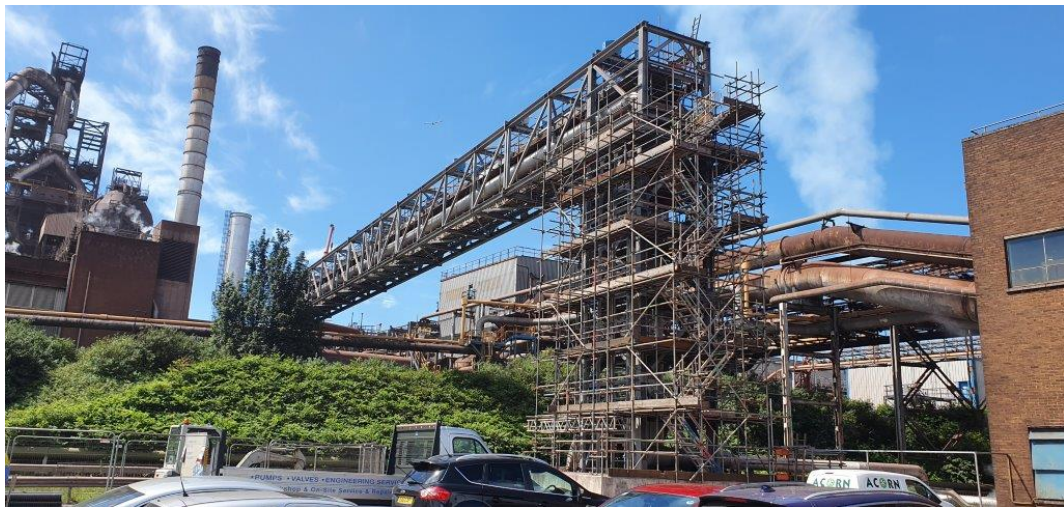
Figure 3.1: View of the Bridge from ground level at the North end of the Bridge, looking South
