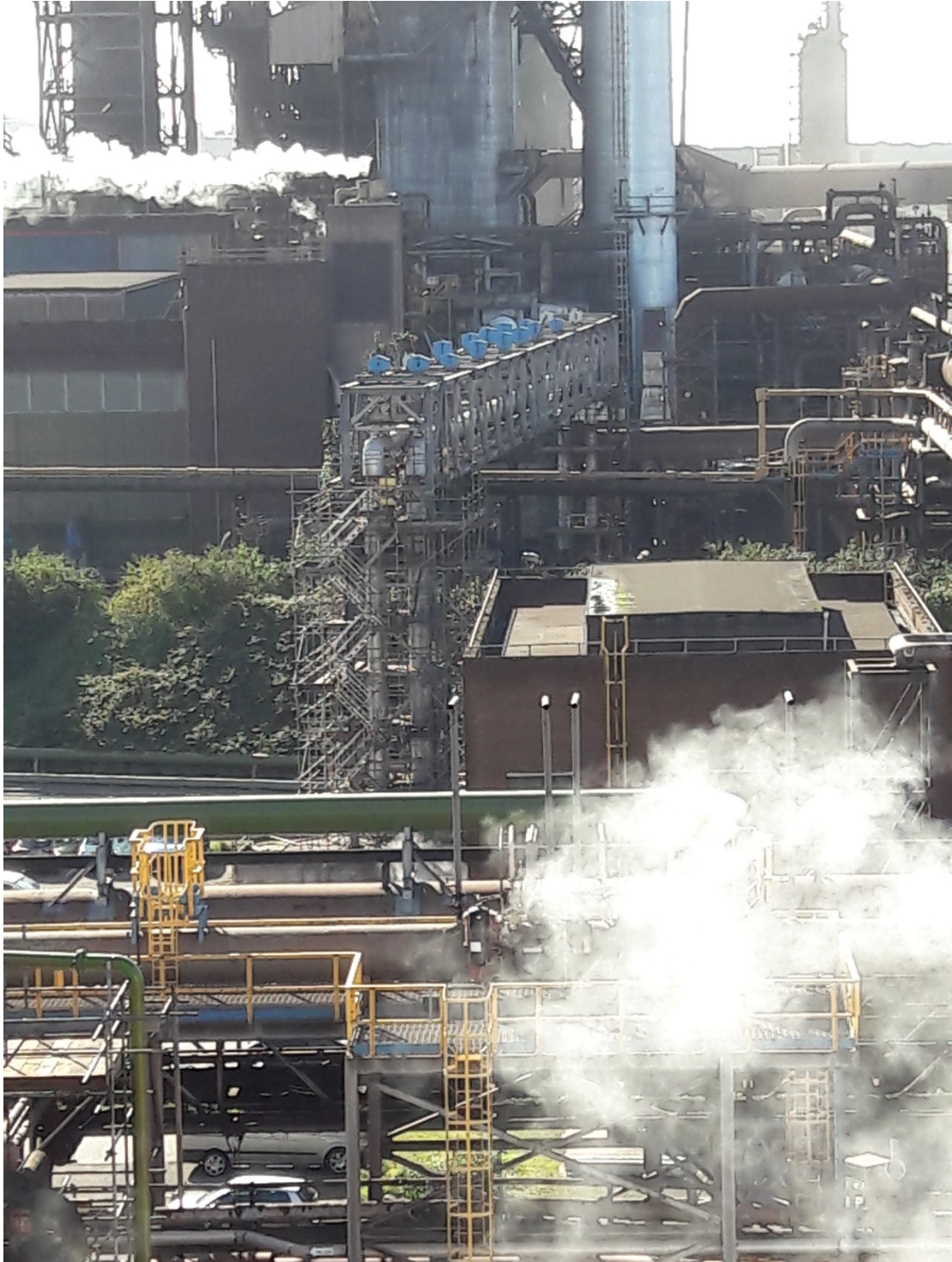
Figure 1.1: Taken from a scaffold tower at Margam C, looking South towards the bridge
