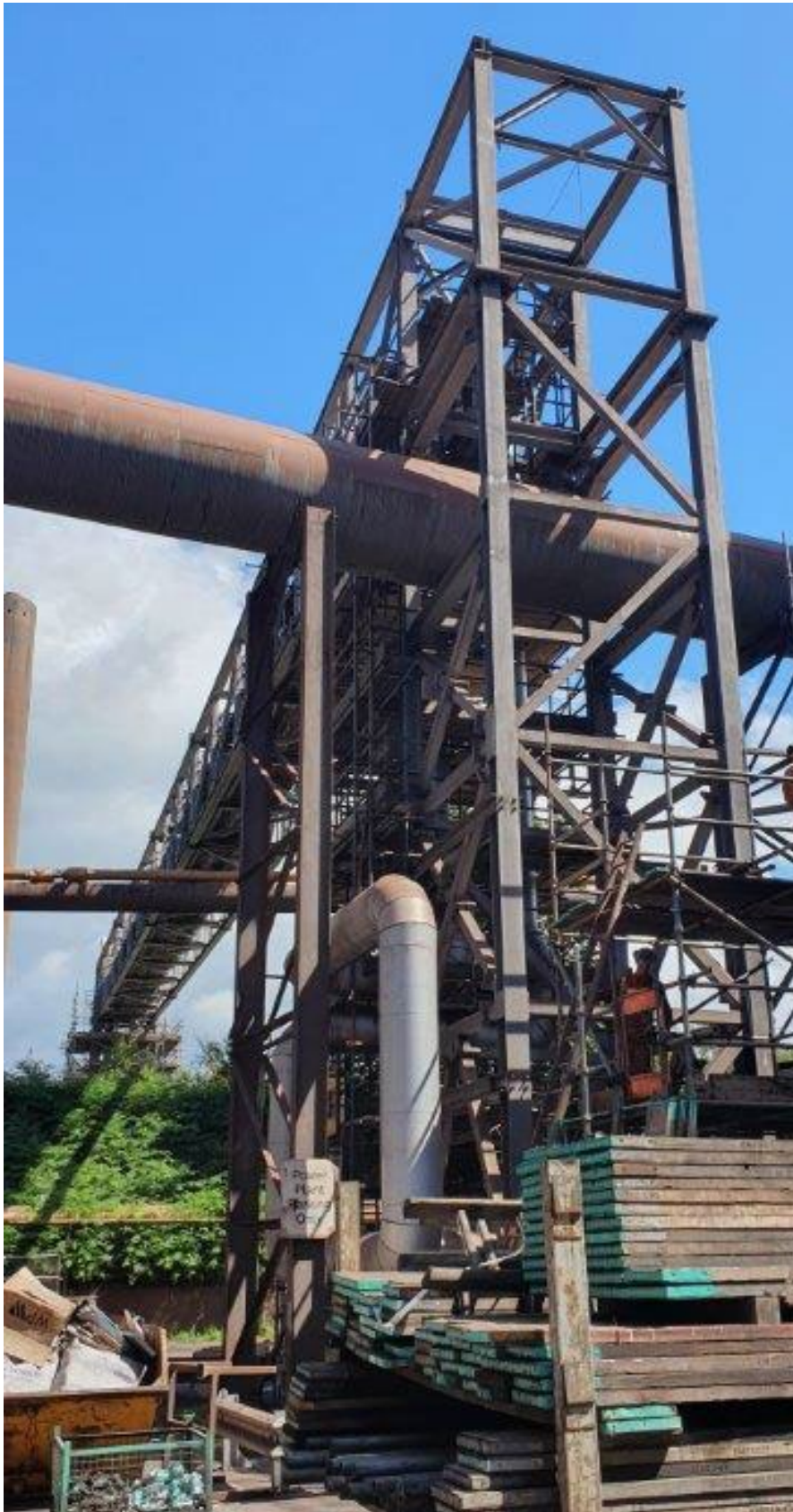
Figure 1.10: Ground level at the South end of the Bridge, looking North
