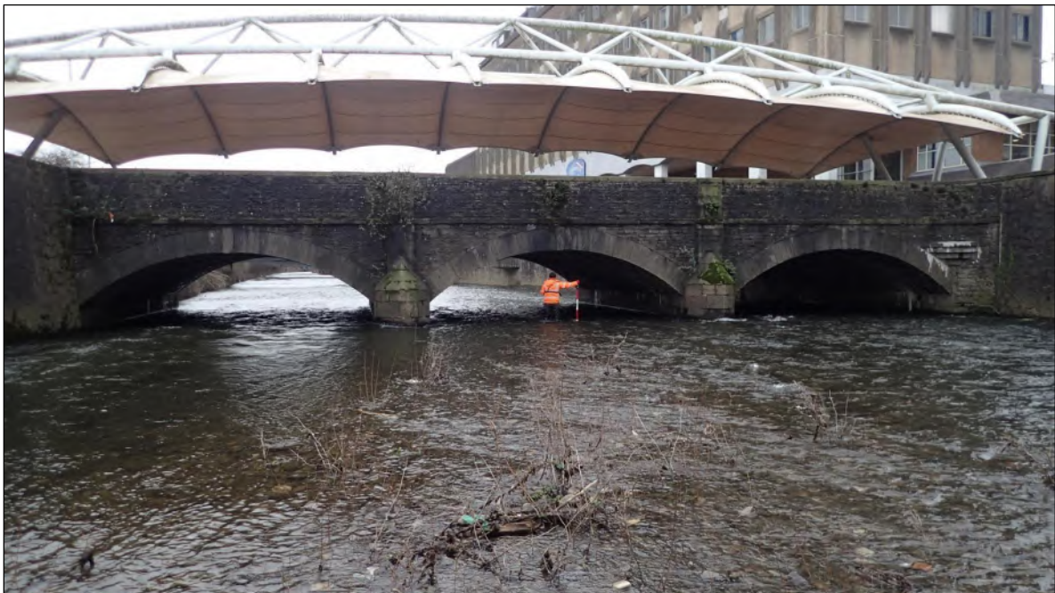
Figure 4-11 Upstream face of the High Street bridge over the River Afan
