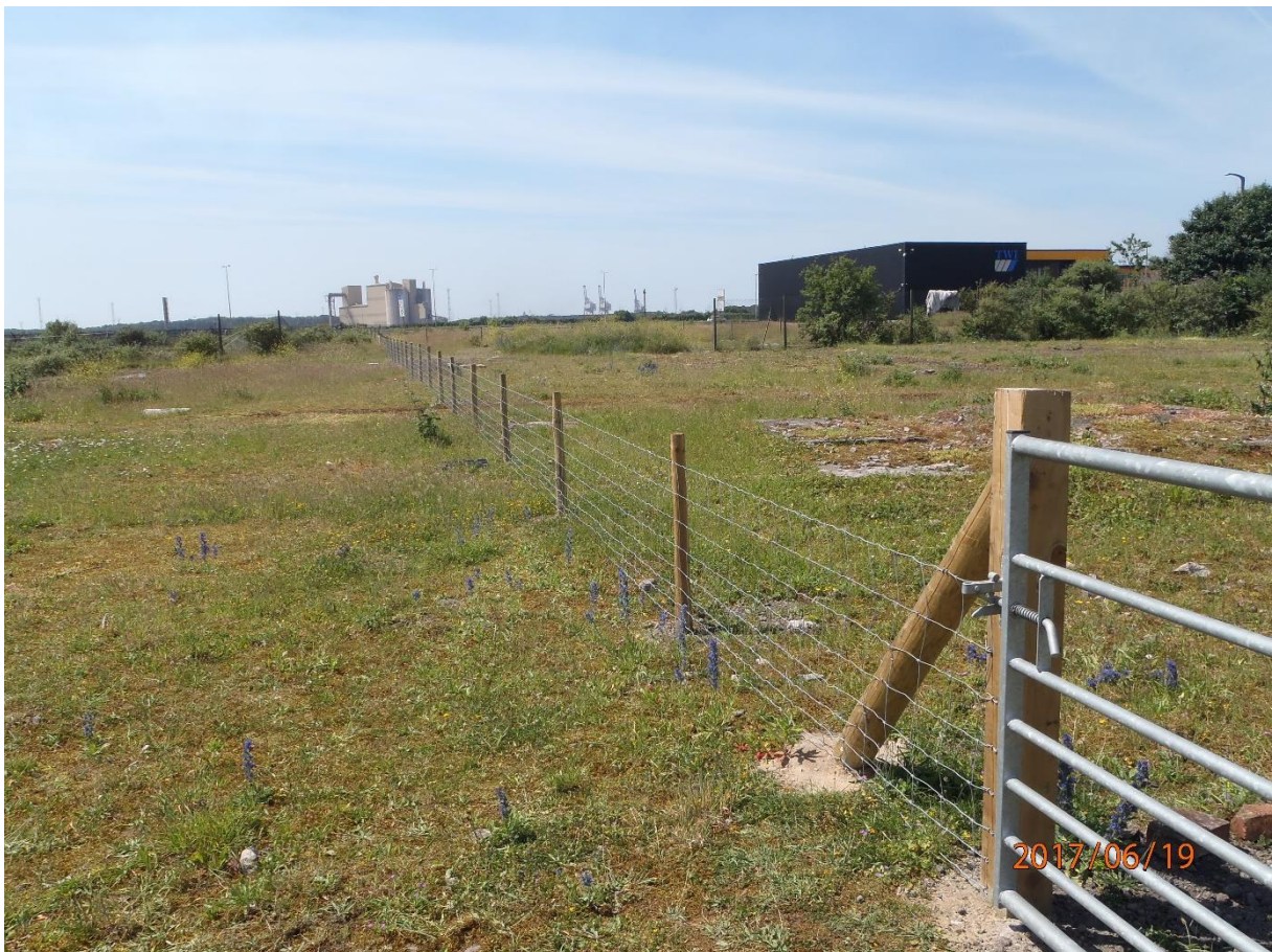
Plate 20: View looking south across site showing recently erected fencing
