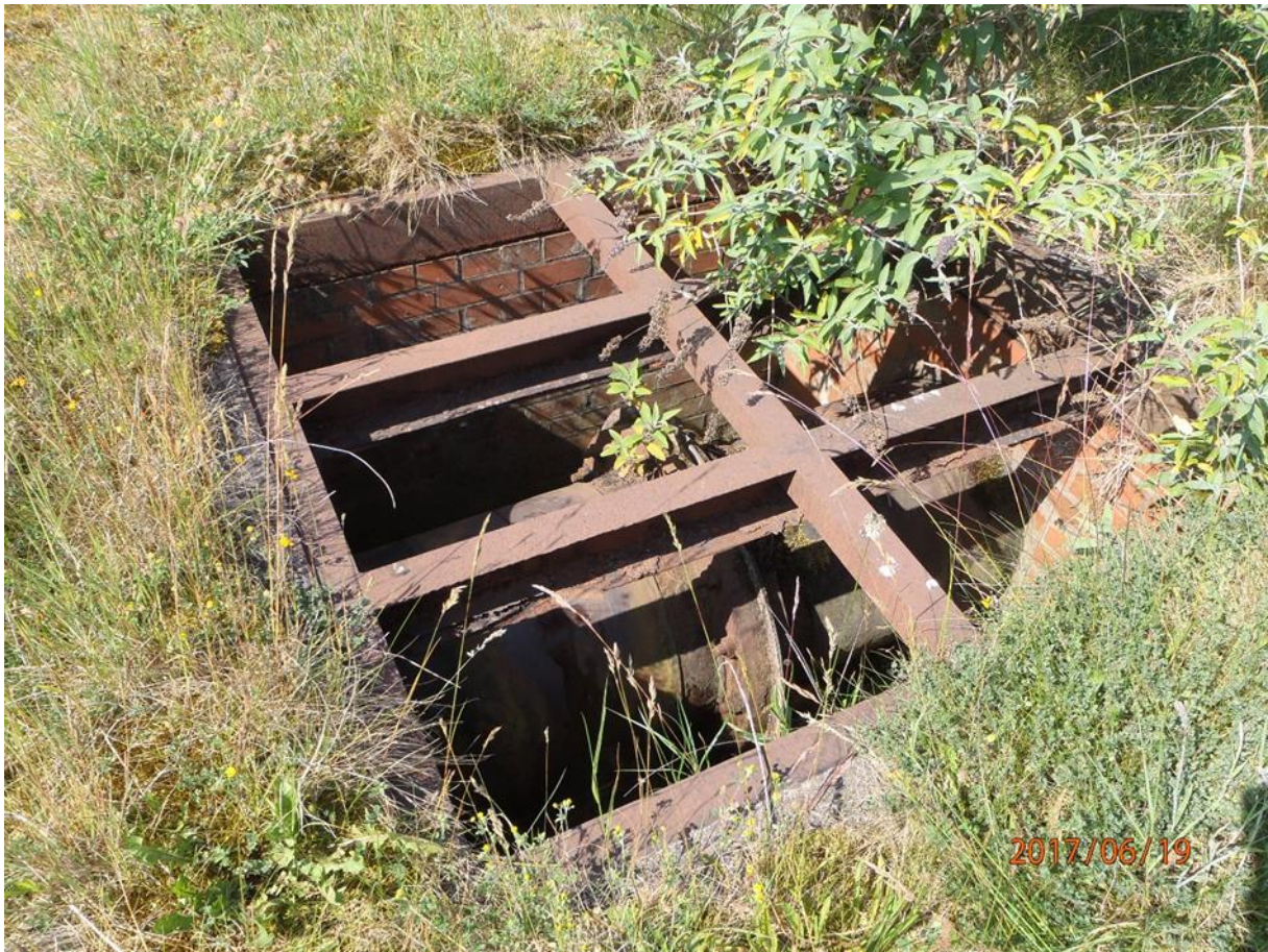
Plate 27: Remains of industrial pipe at south east of the site
