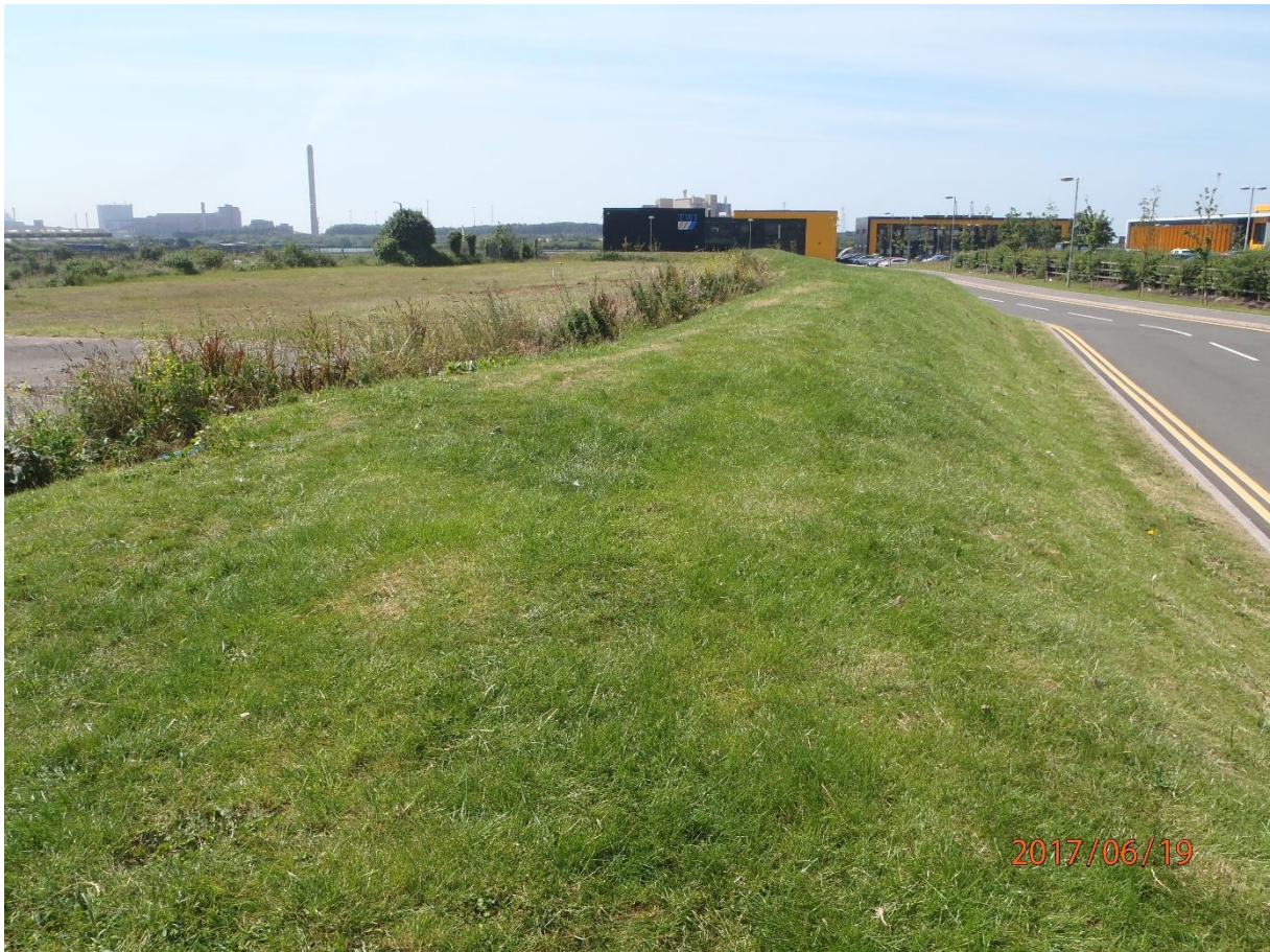
Plate 11: View looking south along western boundary of the site showing earth bund (approx. 2m height)
