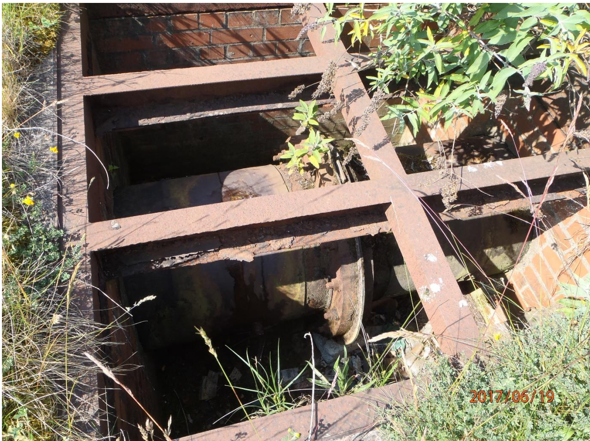
Plate 28: Remains of industrial pipe at south east of the site
