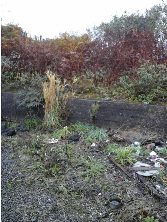
Photo 1: Port Talbot Dock wall, located south west of the site.
