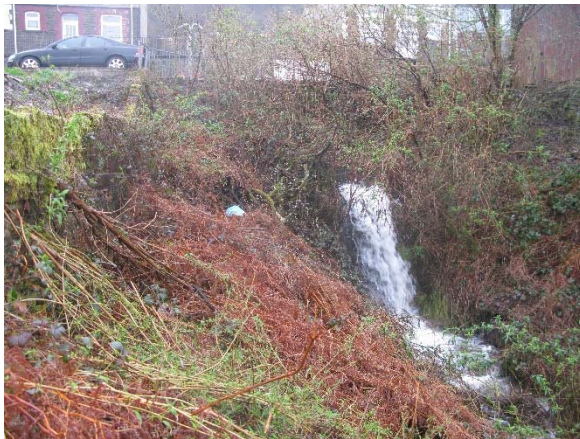
Adjacent tributary of the River Afan just off the eastern site boundary.
