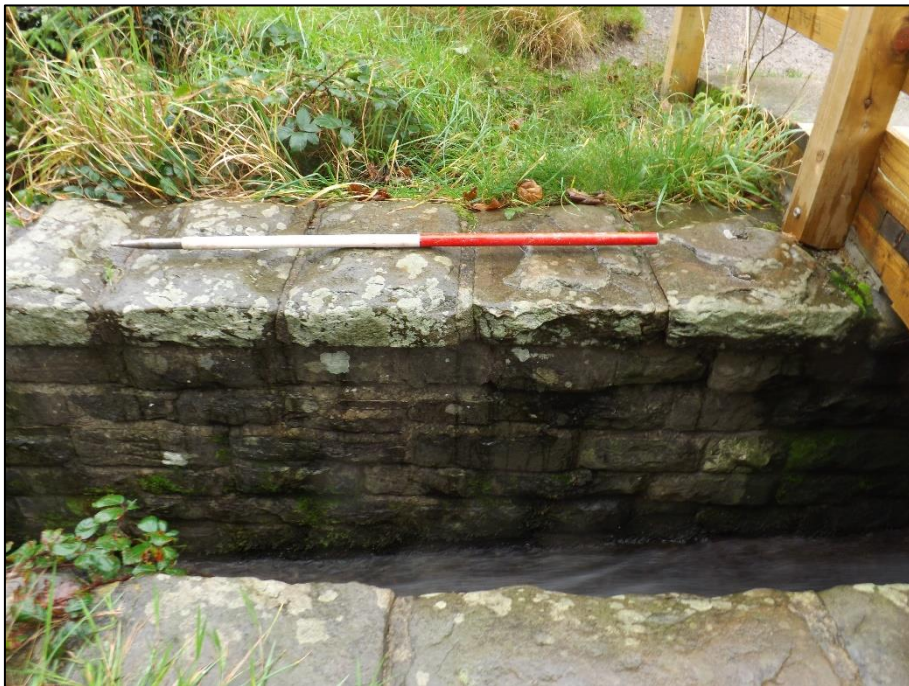
Plate 4. North wall of the spillway channel of Structure 1. This appears to be a later re-build, possibly following insertion of a drainage pipe immediately north. View to north west, scale division 0.5m.
