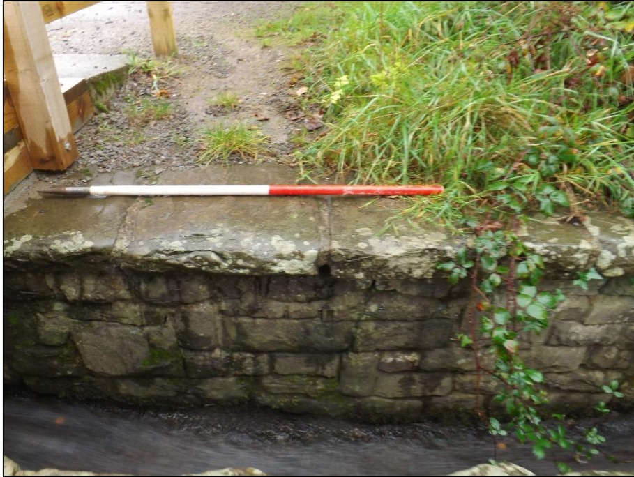
Plate 3. South wall of the spillway channel of Structure 1. This is the original appearance of the masonry in the feature. View to south east, scale division 0.5m.
