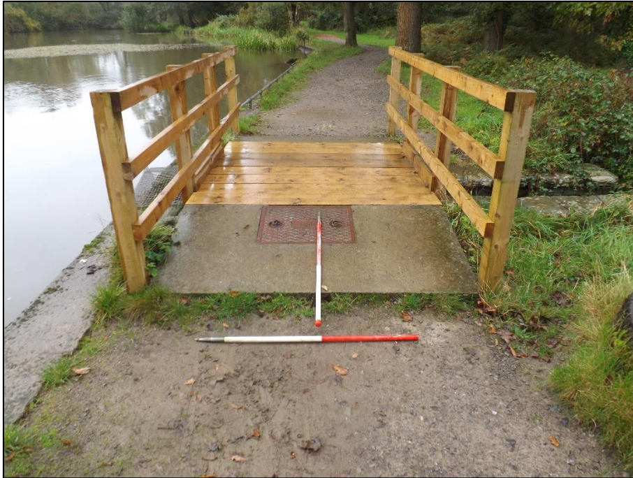
Plate 1. View of the newly constructed footbridge over spillway Structure 1. View to south east, scale divisions 0.5m
