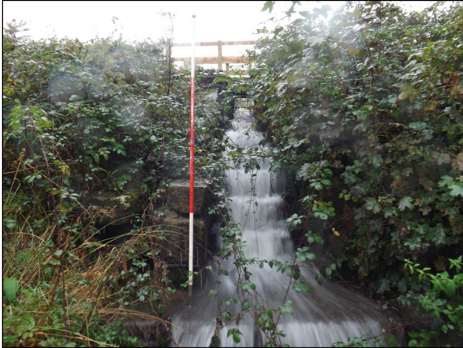
Plate 5. View towards the stepped element of the spillway. A relatively modern drainage pipe is located to the left of the white length of the scale. View to north east, scale is 2m long.
