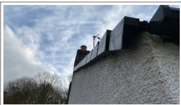
Photo 5: West facing gable end
