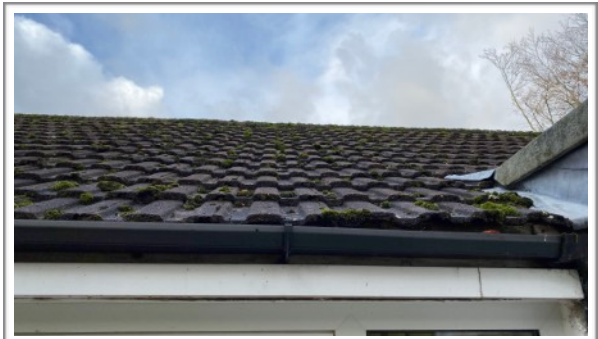
Photo 4: Tight fitting moulded clay roof tiles
