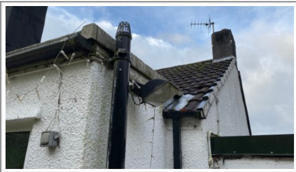
Photo 1: West facing gable end
