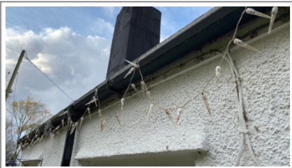
Photo 3: South facing elevation
