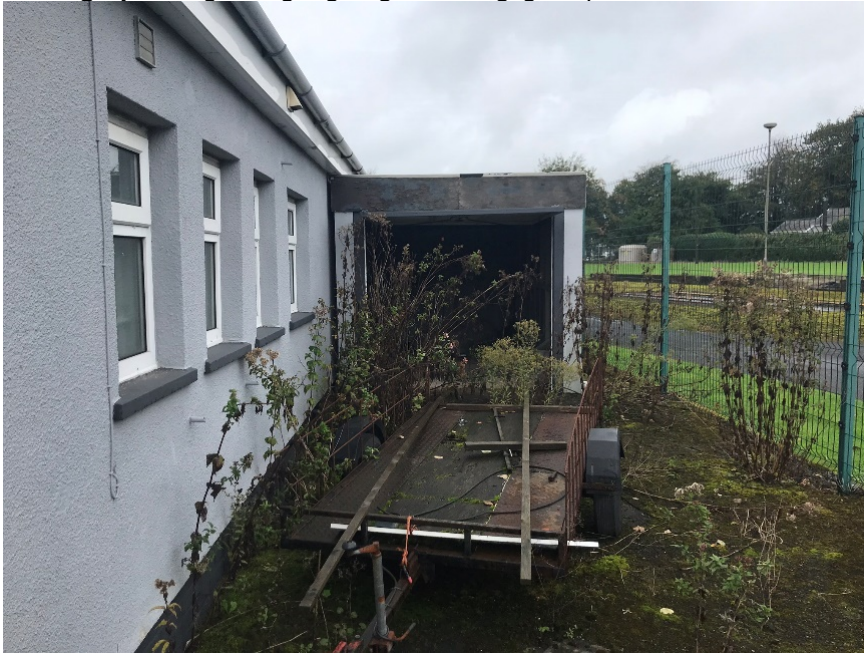
Photograph 3: lightweight garage has negligible potential for bats
