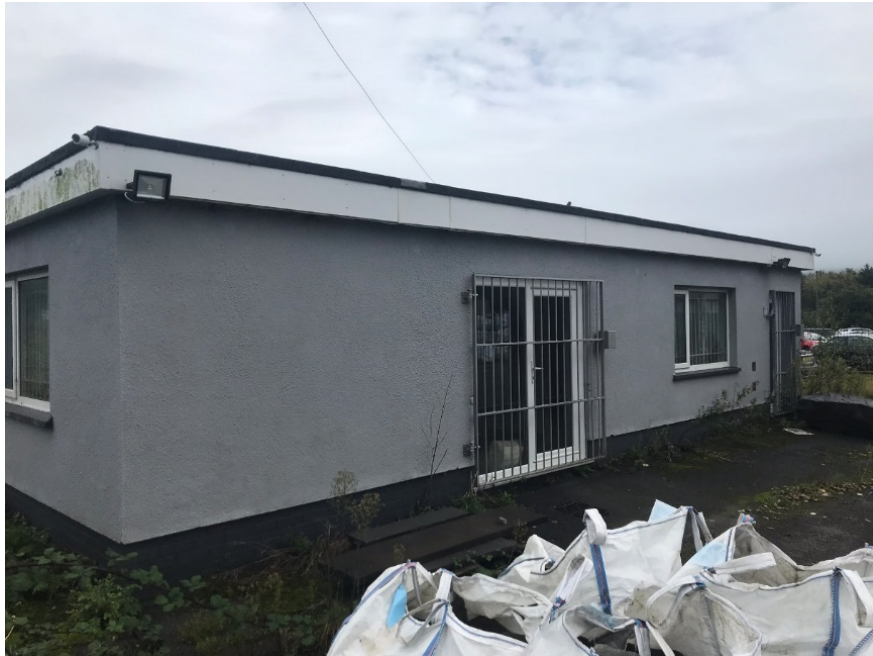
Photograph 1: Single storey building
