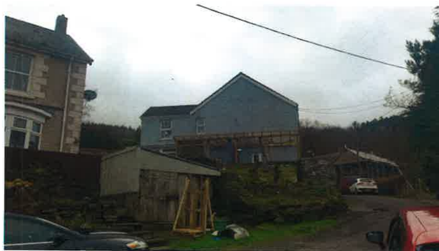
Side elevation & adjacent building/land.
