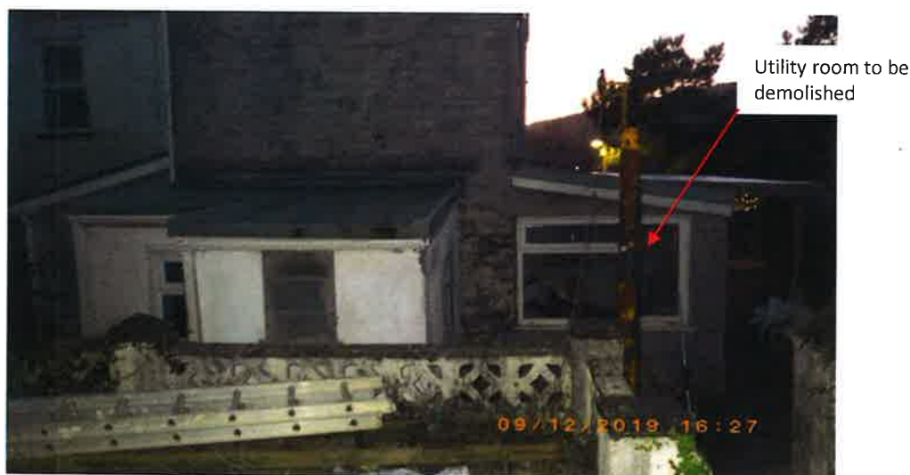
Rear elevation and Utility Room. The latter is to be removed.
