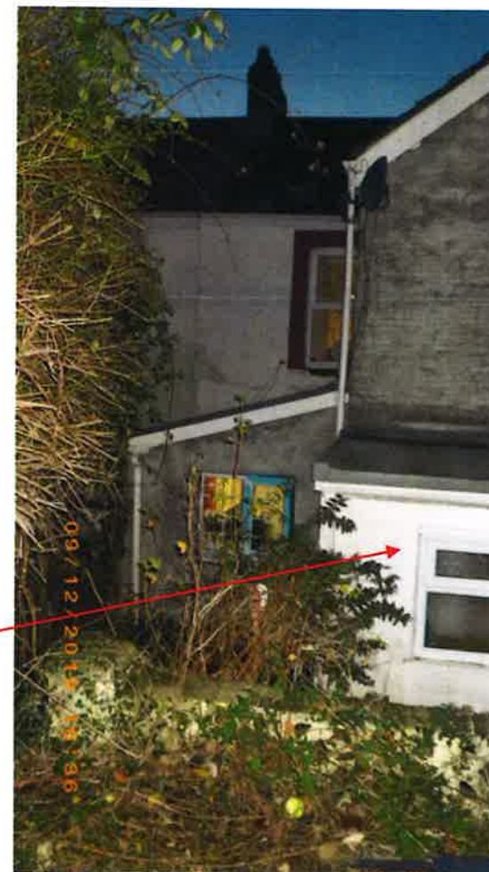
Side elevation and Utility Room. The latter is to be removed.
