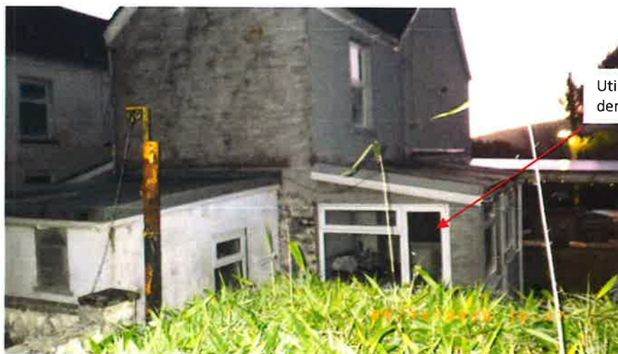
Rear elevation and Utility Room. The latter is to be removed.
