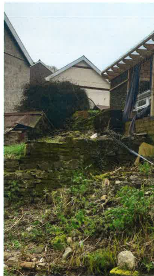
Adjacent building/land – Refer to RED circled area.
