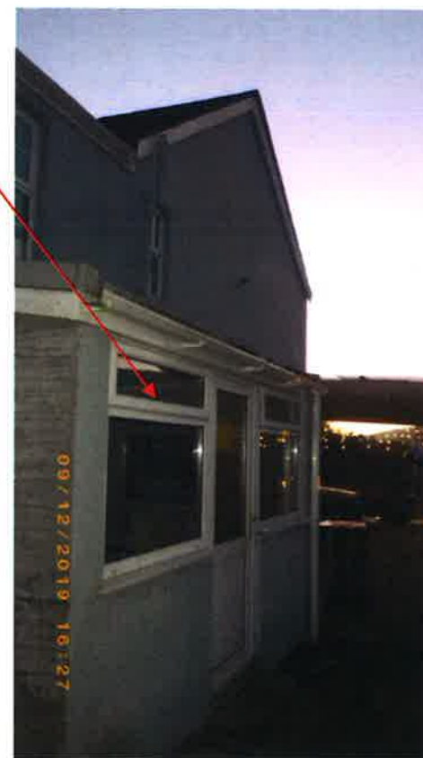
Utility Room to be removed.
